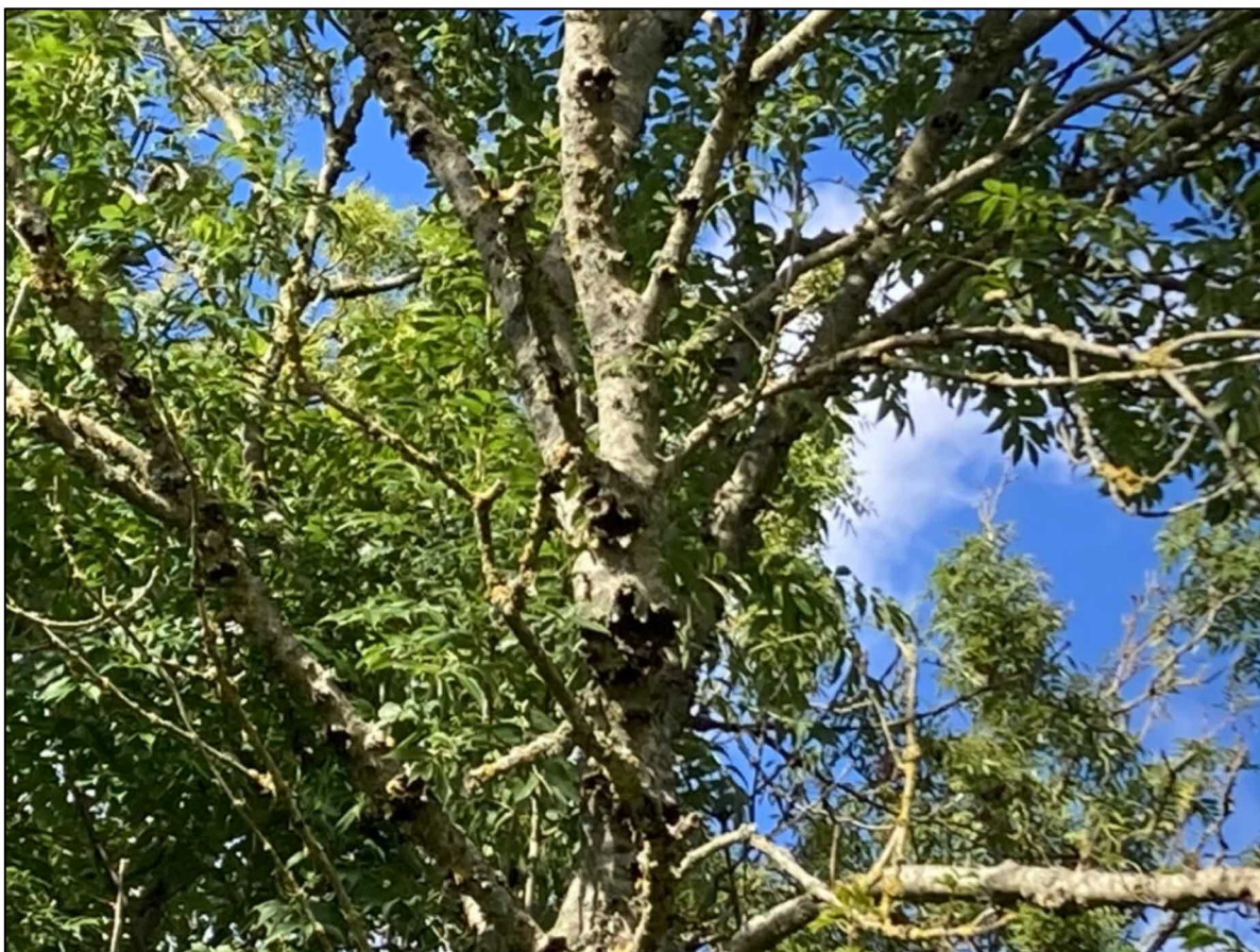
Photograph 6. View of the two cankers on the semi-mature ash tree which have potential to support roosting bats.
