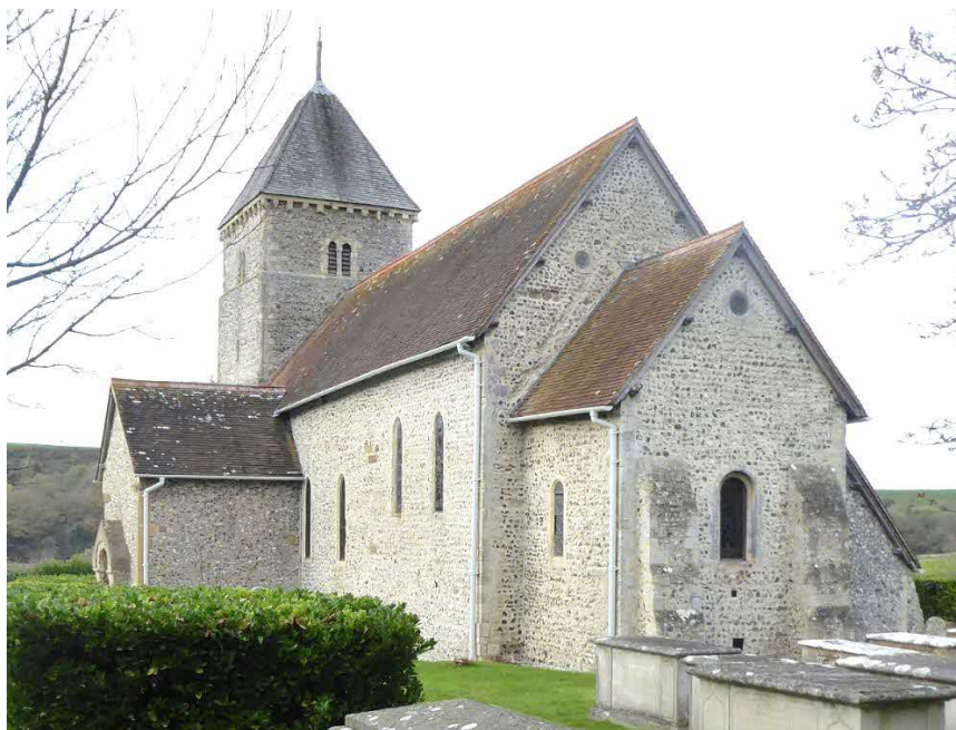
Church from the east, showing sanctuary, and choir as extension of the nave
