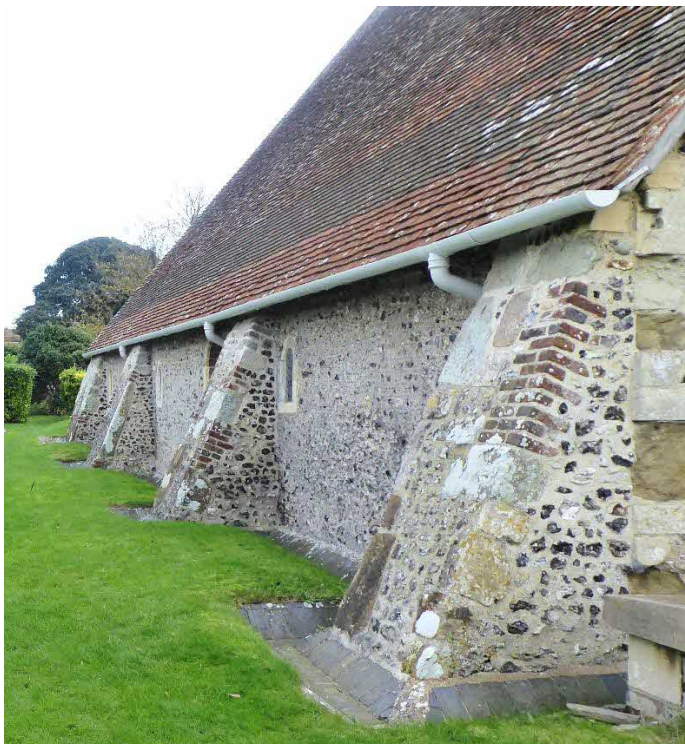
The 12 th C north aisle with later buttresses
