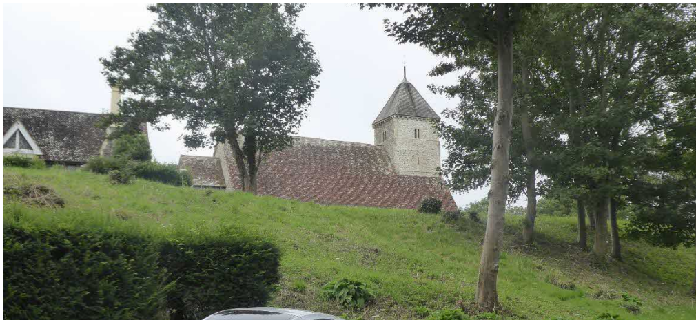
Top: view from north of Green at present, and, below, with the extension
