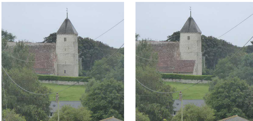
Long view from north, with photomontage on the right showing the extension
