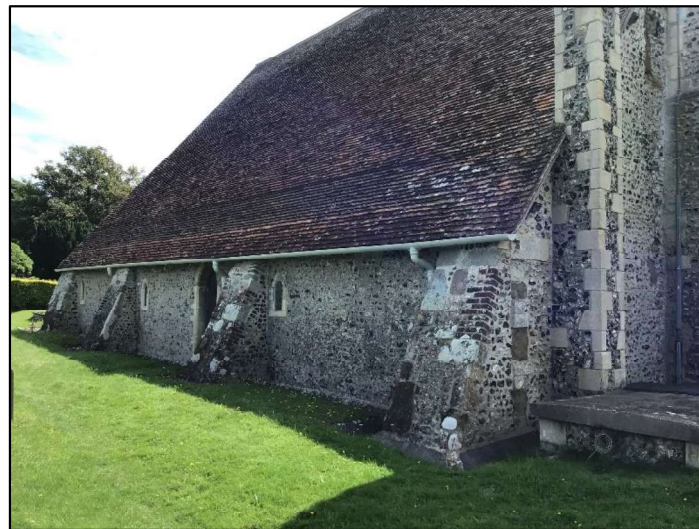
Fig. 3: The north aisle (note blocked window to left of western buttress)
