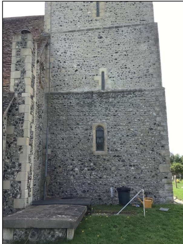
Fig. 8: North wall of tower
