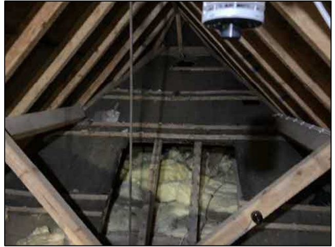
Photograph 6a (left) & 6b (right). Left – View of internal guttering in the loft void, which provides gaps. Right – View of the bitumen felt and crossbeams separating the main and connecting voids, and the gap present close to the floor.
