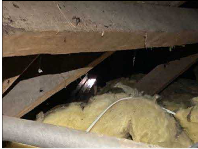
Photograph 6a (left) & 6b (right). Left – View of internal guttering in the loft void, which provides gaps. Right – View of the bitumen felt and crossbeams separating the main and connecting voids, and the gap present close to the floor.
