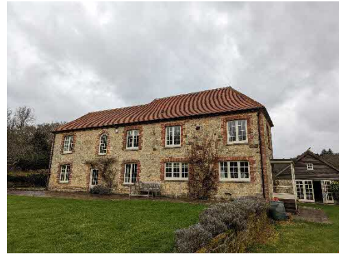
Figure 6 – Existing extension has a higher roof than the main house
