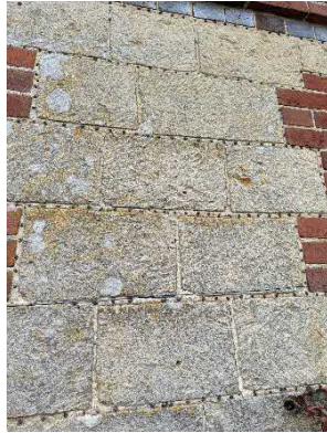
Figure 5 – Existing flint galletting in the Wealden Sussex sandstone wall
