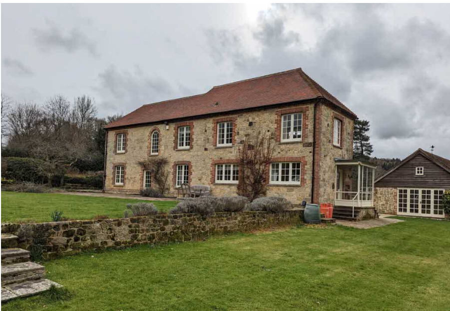
Fig. 3 – East Elevation. Clearly demonstrating the higher ridgeline to the 1960s/1970s extension to the north and original house to the left-hand side.
