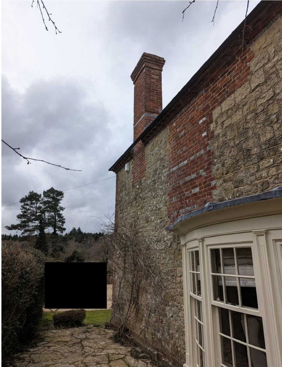
Fig. 4 – South Elevation. With later bow window on the site of former fireplace. Assumed to have been completed in the 1960s/1970s.
