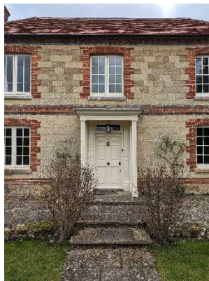
Figure 7 – Existing timber porch proposed to be replaced
