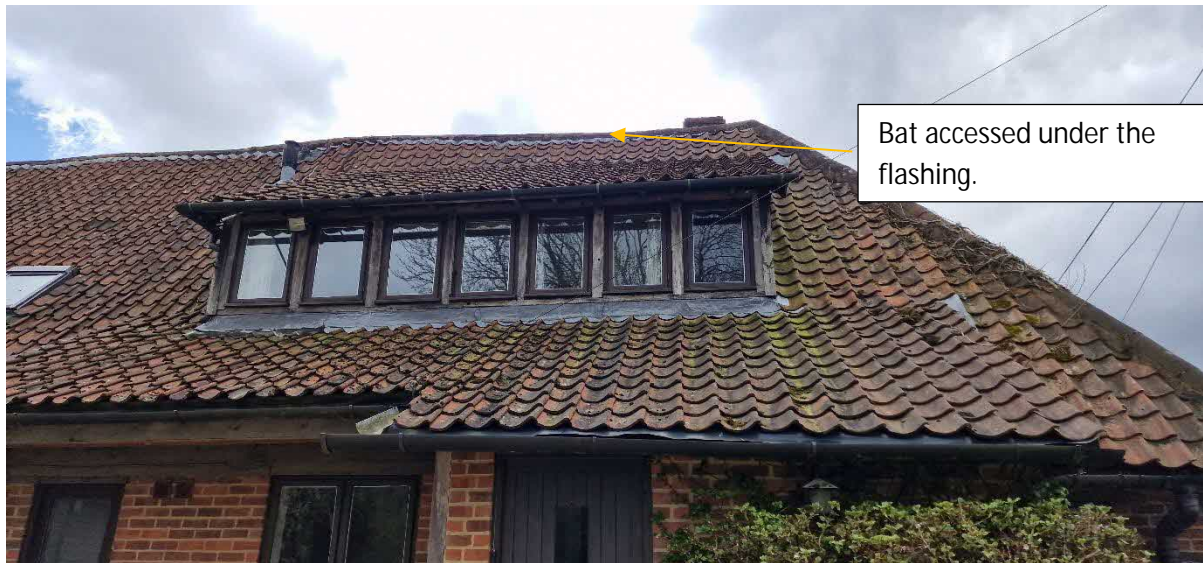
Picture 1: Looking at the front of building 1 showing the dormer window
