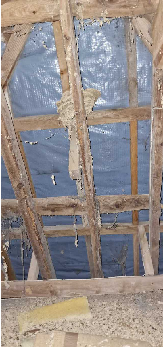
Picture 7: Showing the roof membrane in roof void 1
