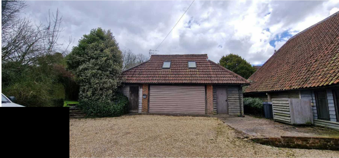
Picture 5: Showing the western elevation of building 2
