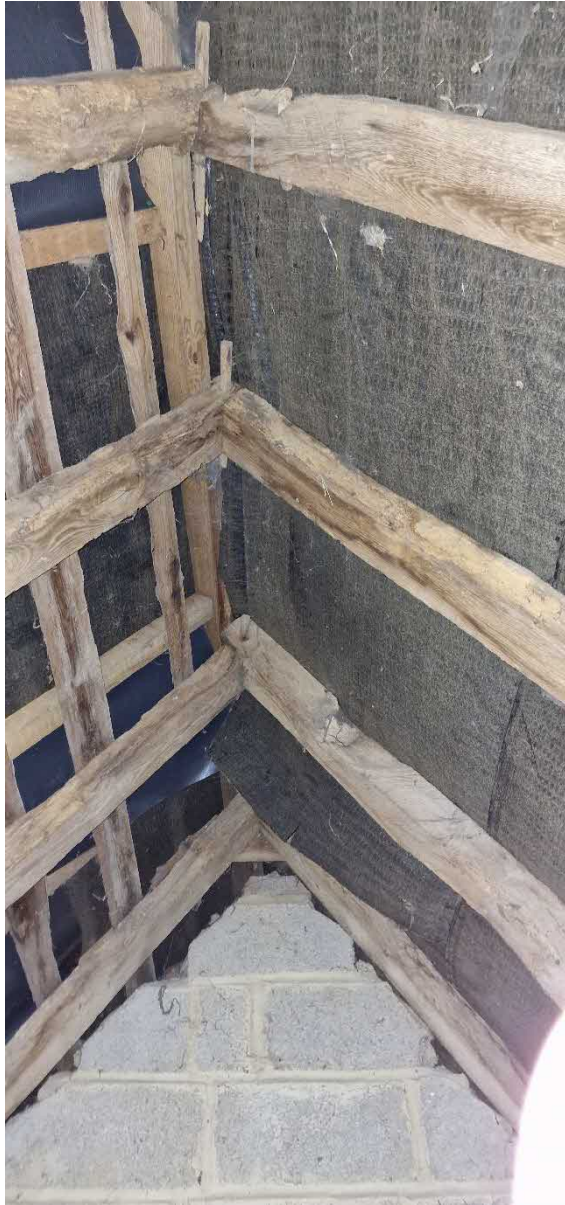
Picture 8: Showing the roof membrane in roof void 2
