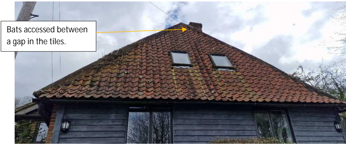
Picture 3: Showing the north-western elevation. (Building 1)
