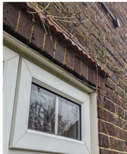
3. Bricks to match the existing house will be utilised for new walls Existing details will be replicated in a contemporary way for the rear extension the tile cavity tray amended to a steel overhang to define the opening
