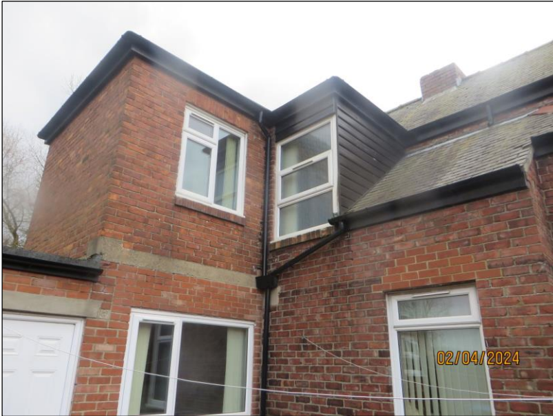
Figure 14. Northern facing elevations, showing different roofing structures.
