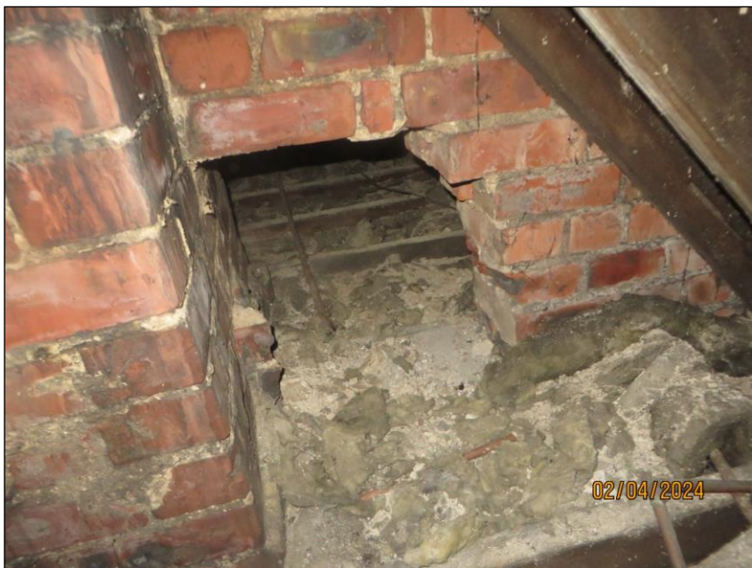
Figure 19. Access gap between the two loft voids.
