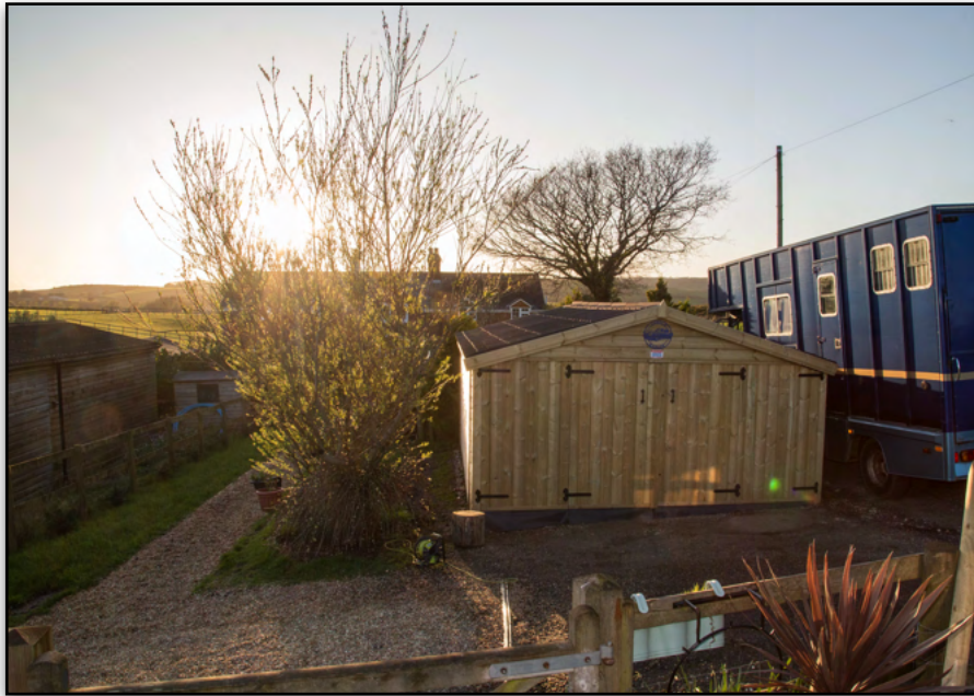
Front wide view. Dwelling houses 30m in the background. Neighbours stables to the left / south
