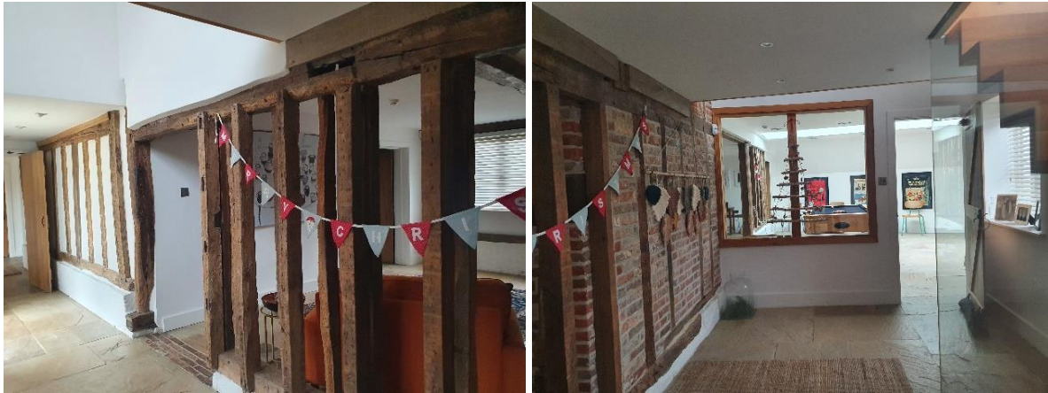
Timber frame corridor
