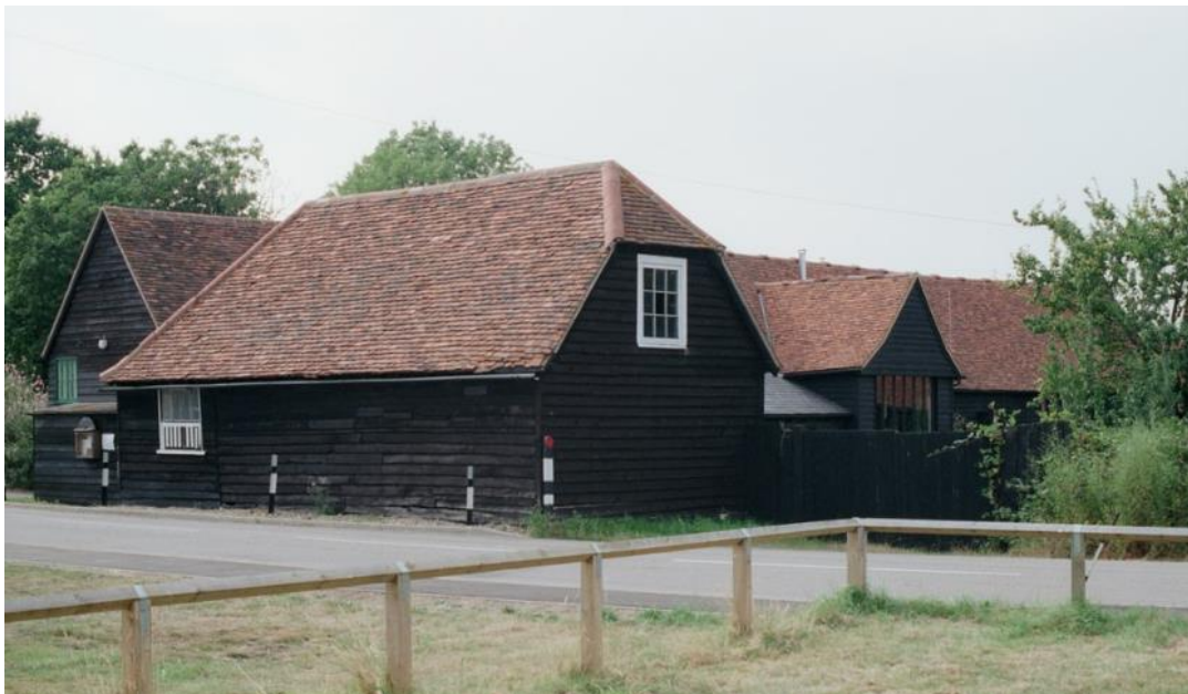
Farm buildings and village hall at Fanshaws farm
