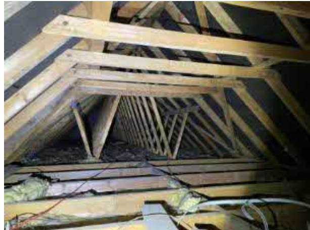
Plate 22: Roof void - structure 4 (above single storey) extension.
