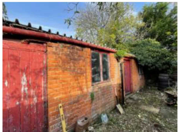
Plates 9 and 10: Brick outbuilding (former coach house) to north of main pub complex: showing corrugated metal roof and glazed windows (Figure 3, structure 5).
