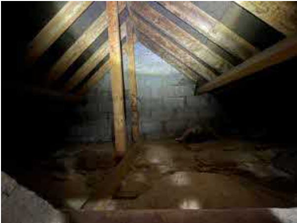
Plate 21: Roof void - structure 3.
