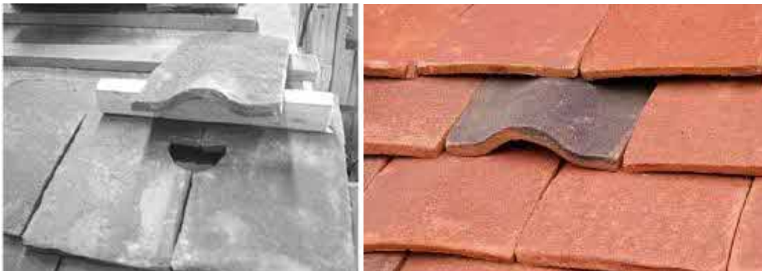
Figure A6.2. Roof slope crevice roost bat access tile suitable for areas of clay tiling. Bespoke lead access tiles can also be used.
