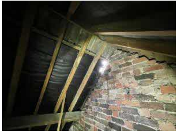
Plates 15-16 Roof void – structure 1: showing roof timbers, brick gables and roof linings.
