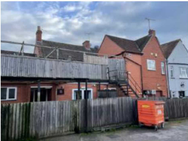
Plate 7: Western elevation; showing the two-storey extensions (structures 2 and 3, Figure 3) and single-storey extension with a flat roof (structure 4, Figure 3) and adjoining wooden canopy.
