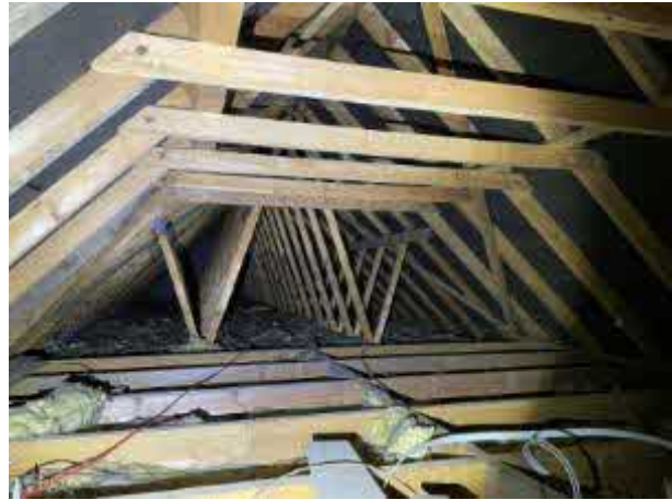
Plate 22: Roof void - structure 4 (above single storey) extension.
