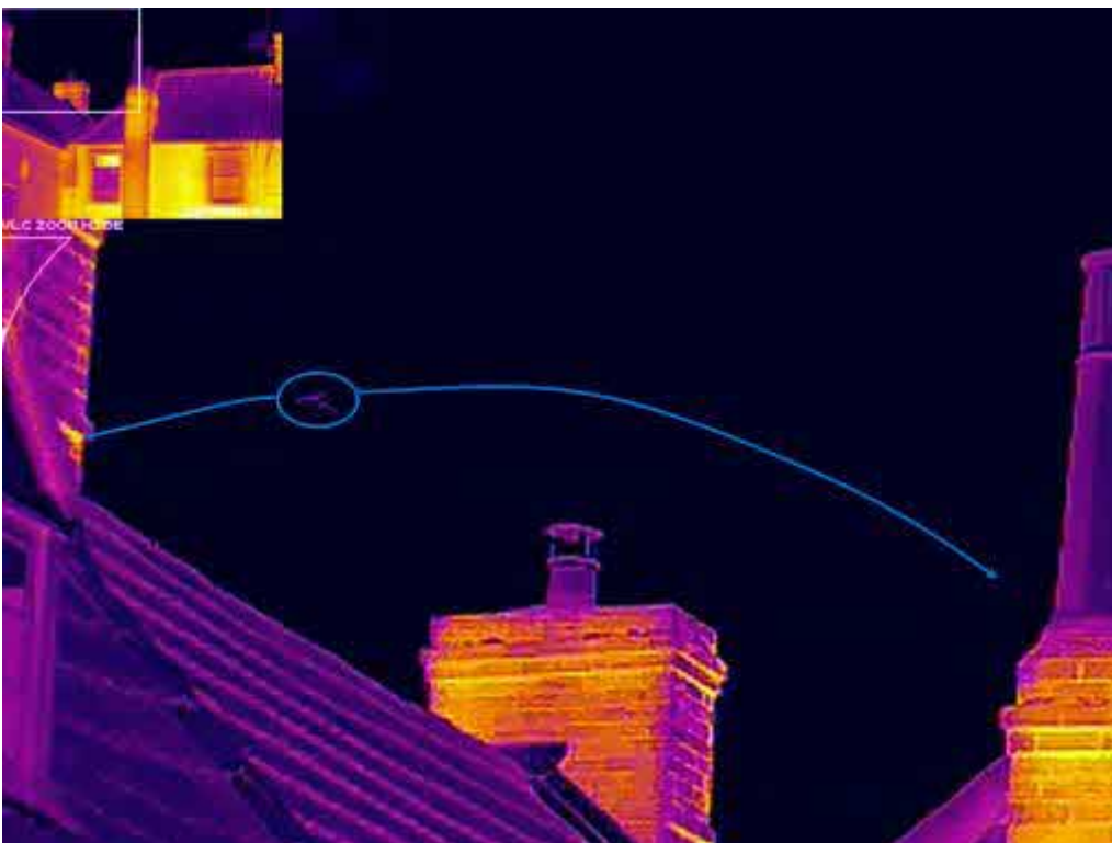
Plate 26: Still from thermographic video showing the flight path of an emerging common pipistrelle from near the base of the east chimney on the south roof, at 2134 on 25 th July 2023. The video clip is available on request.
