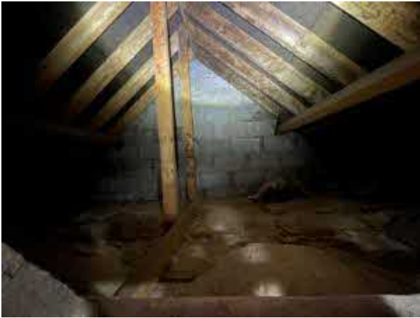
Plate 21: Roof void - structure 3.
