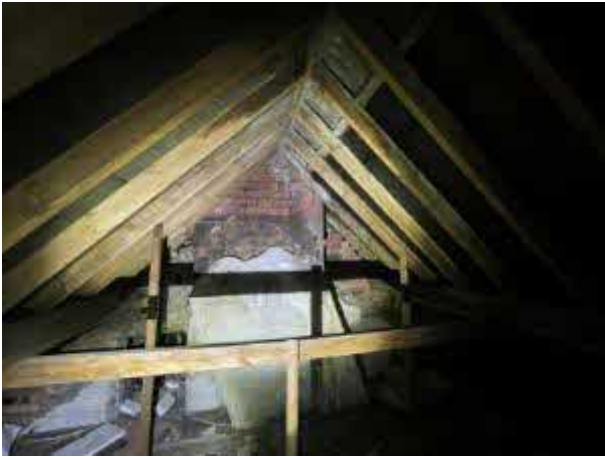
Plates 15-16 Roof void – structure 1: showing roof timbers, brick gables and roof linings.
