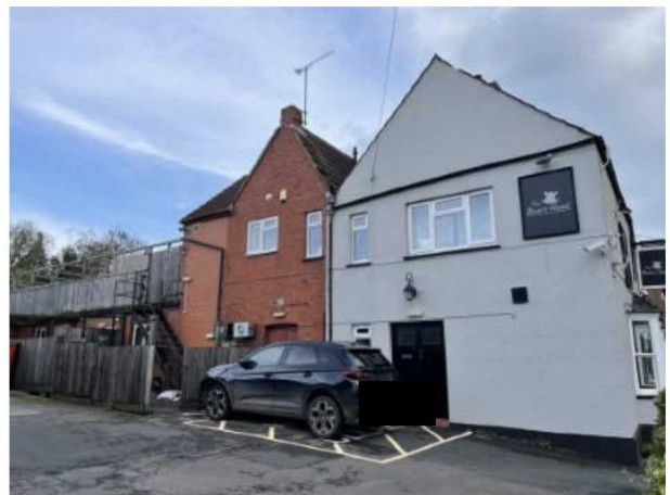
Plates 1 and 2: The Boars Head; showing southern elevation (left) and western gables (right) of structures 1 and 2 (see Figure 3), with pitched, tiled roofs and brick chimneys.
