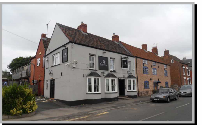
The Boars Head Inn and the adjoining residential unit.
