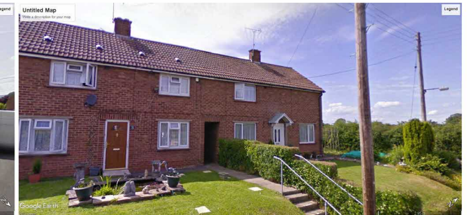
Door canopy covering.
