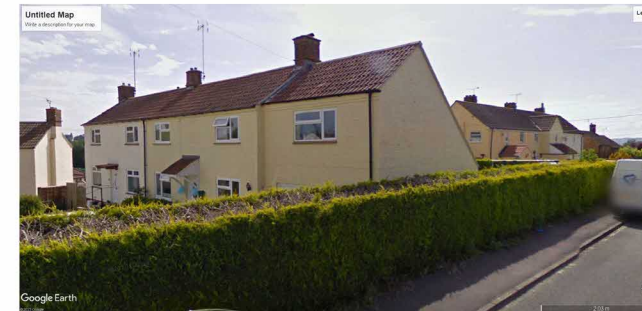
House with cat slide roof to the rear.
