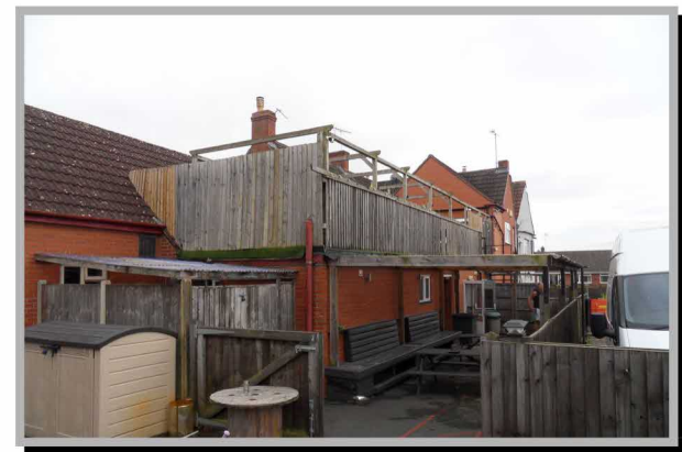
Images to the rear buildings to the Boars Head Inn.
