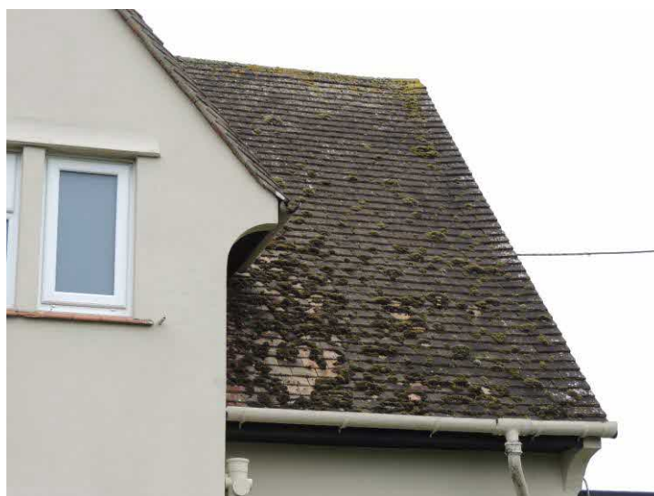
Photo 9: There was a tight seal to the roof tiles
