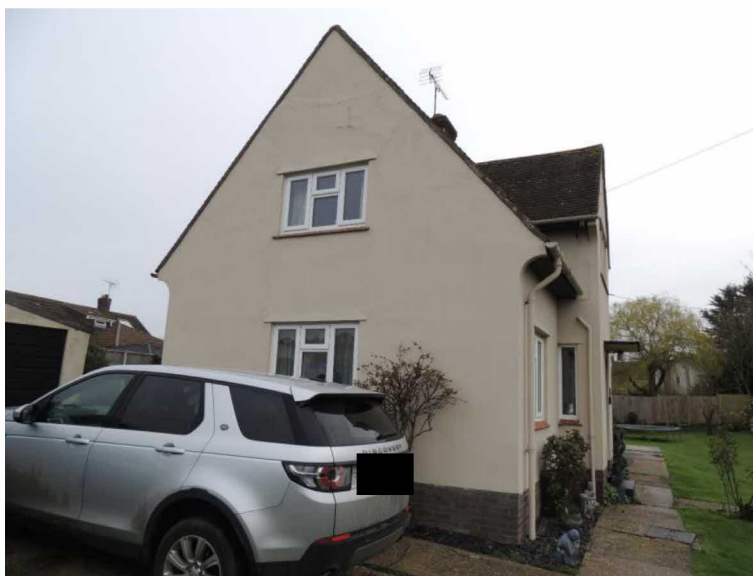
Photo 2: South-western elevation. Note tight seal to gable
