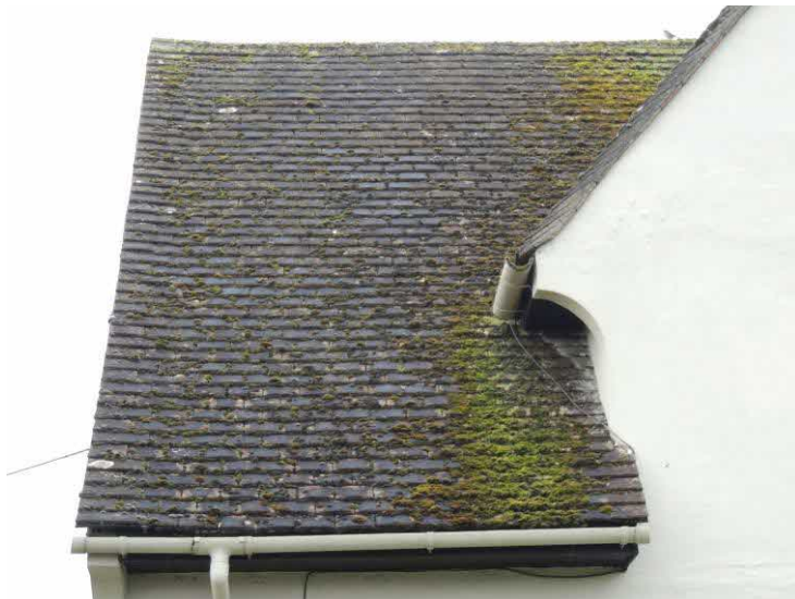
Photo 8: There was a tight seal to the roof tiles
