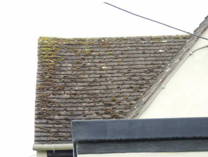
Photo 10: There was a tight seal to the roof tiles
