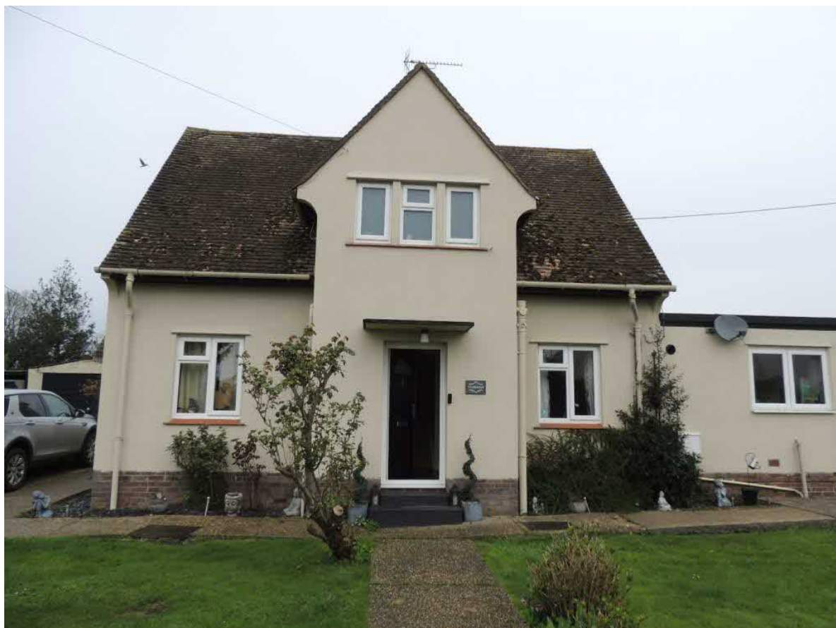
Photo 1: South-eastern elevation. The proposal is to demolish and replace with three new dwellings at the site
