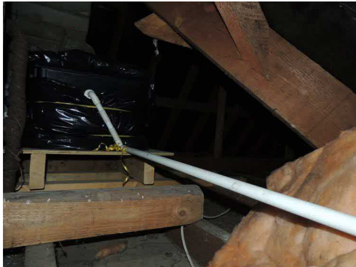
Photo 5: There was no evidence of bats in the loft
