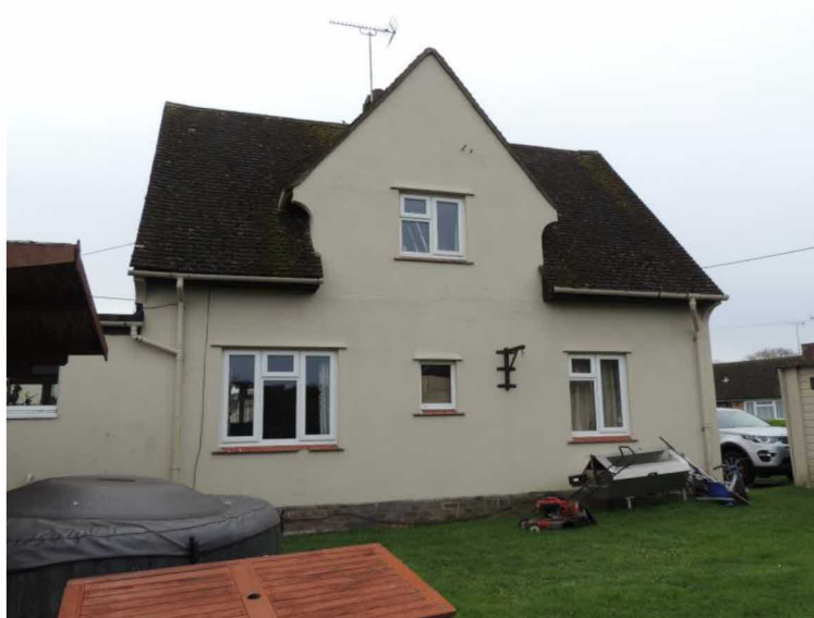
Photo 3: North-western elevation. Note tight seal to gable
