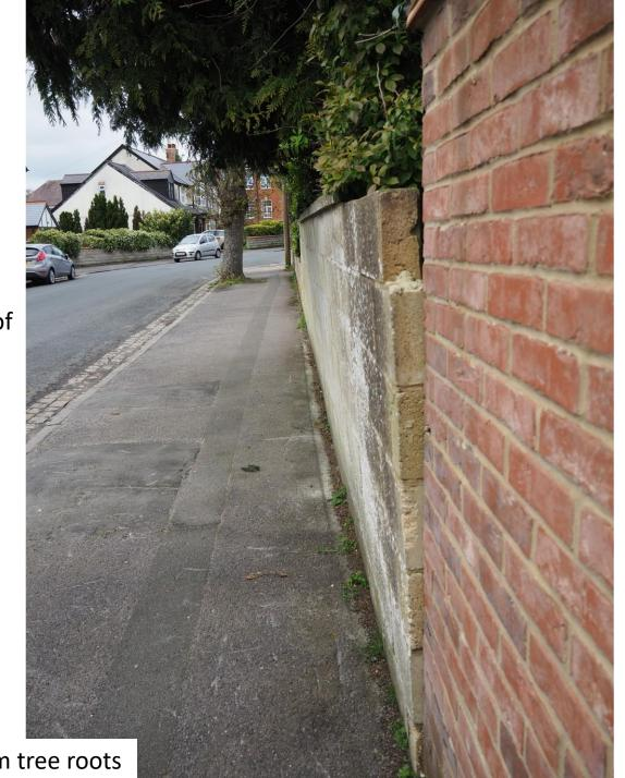
Figure 3 Displacement of wall from tree roots
