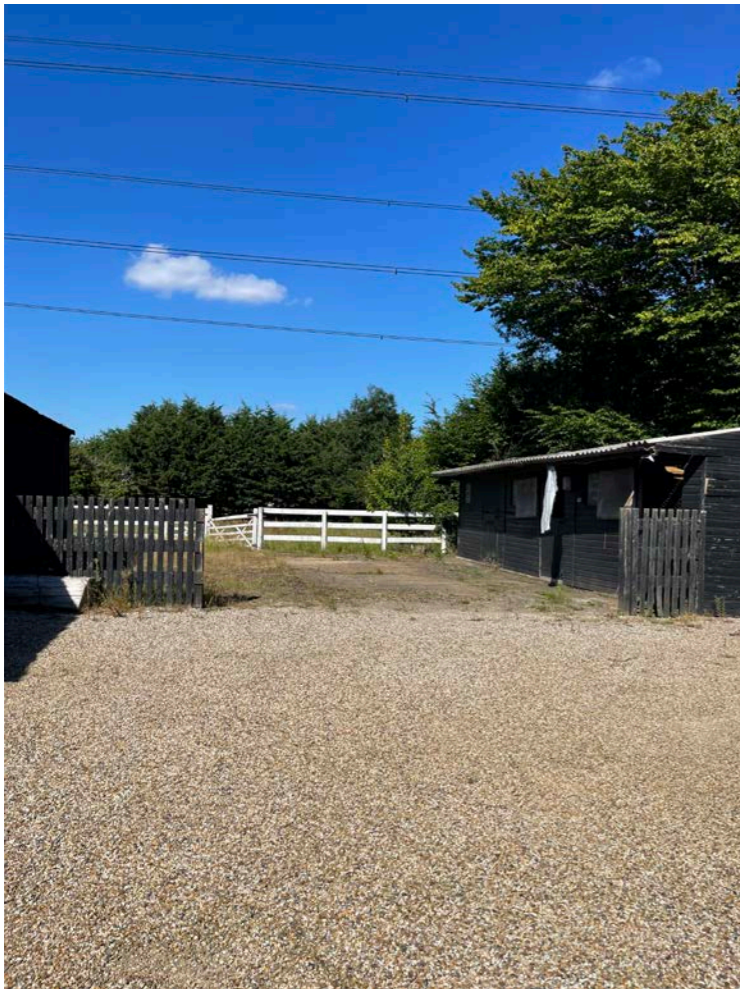
The existing Stable Block
