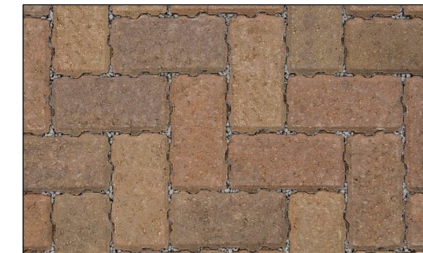
Marshalls Keyblok in Bracken and laid herringbone.
