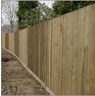
1 Close boarded timber fence around car park and to rear of building, 1800mm high.
