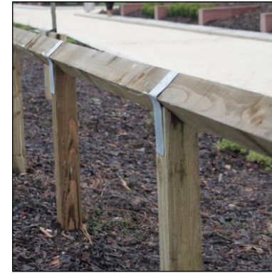
4 Timber Knee Rail with 100mm wide zinc straps. Located along perimeters of soft landscaping
