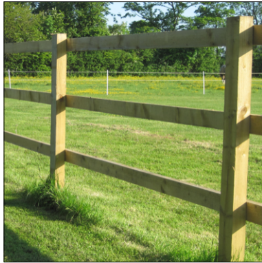
6 Timber Post and Rail Fence, 1200mm high.
