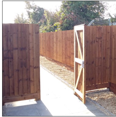
2 Lockable gate with emergency push pad
