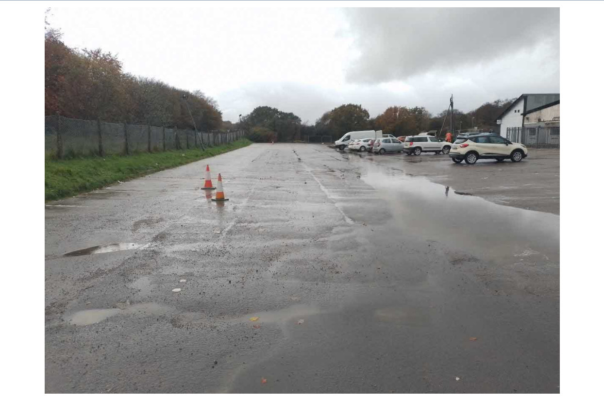
Photograph 2 – Car park area
