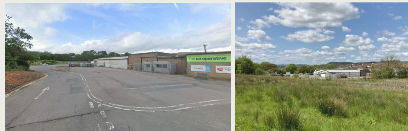
(Left) Street view image within the east site boundary. (Right) Site visit photo showing the view of site from the fields south-east of the existing site boundary.
