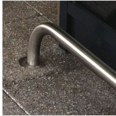
1 Brushed stainless steel low level shopfront protection rails
