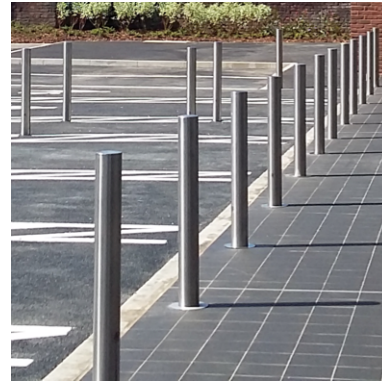
3 Autopa Ltd stainless steel anti-ram bollards, 900mm high above ground, located to front of store between car park and public realm
