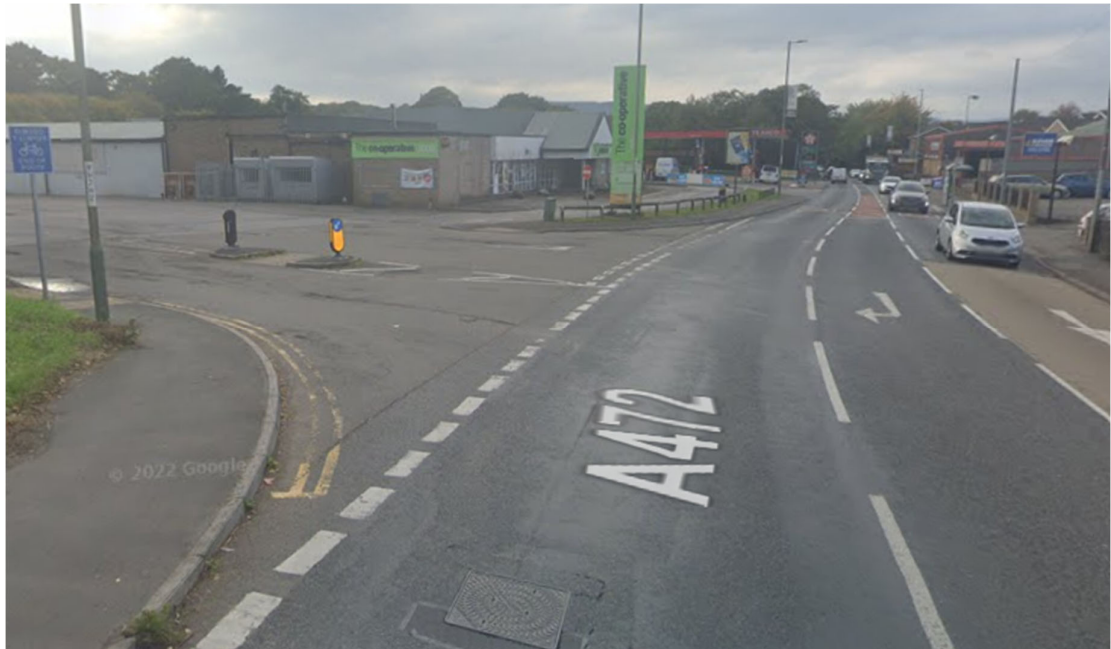
Figure 2.4 - Existing Access from Mafon Road
