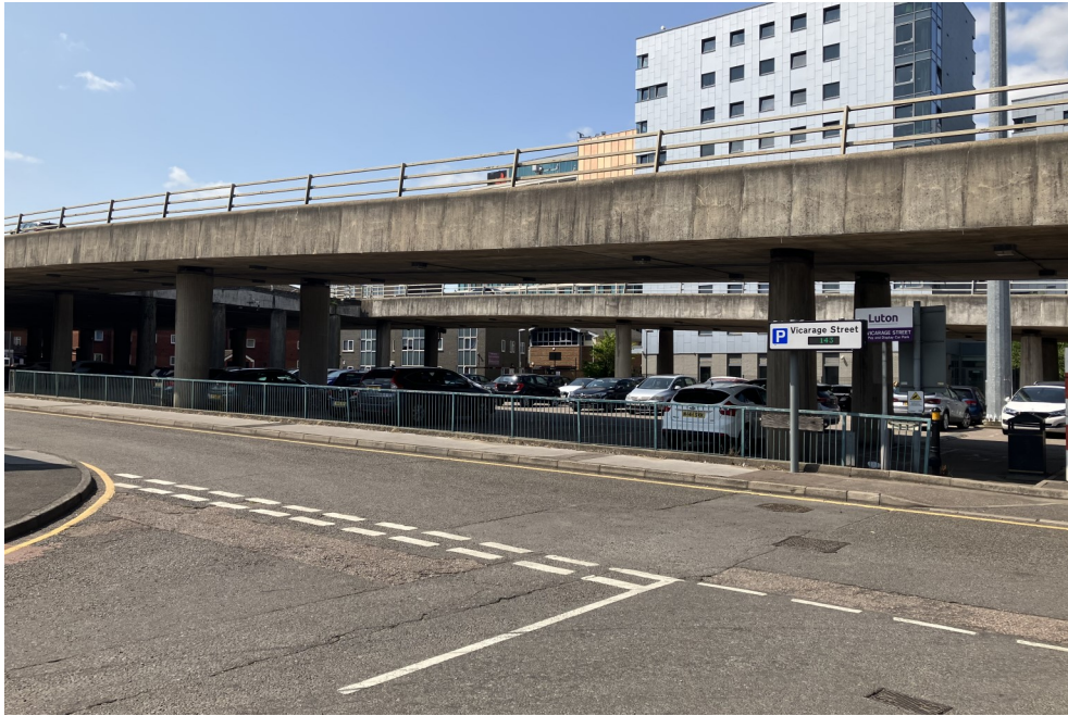
Site area looking northwest towards elevated A505
