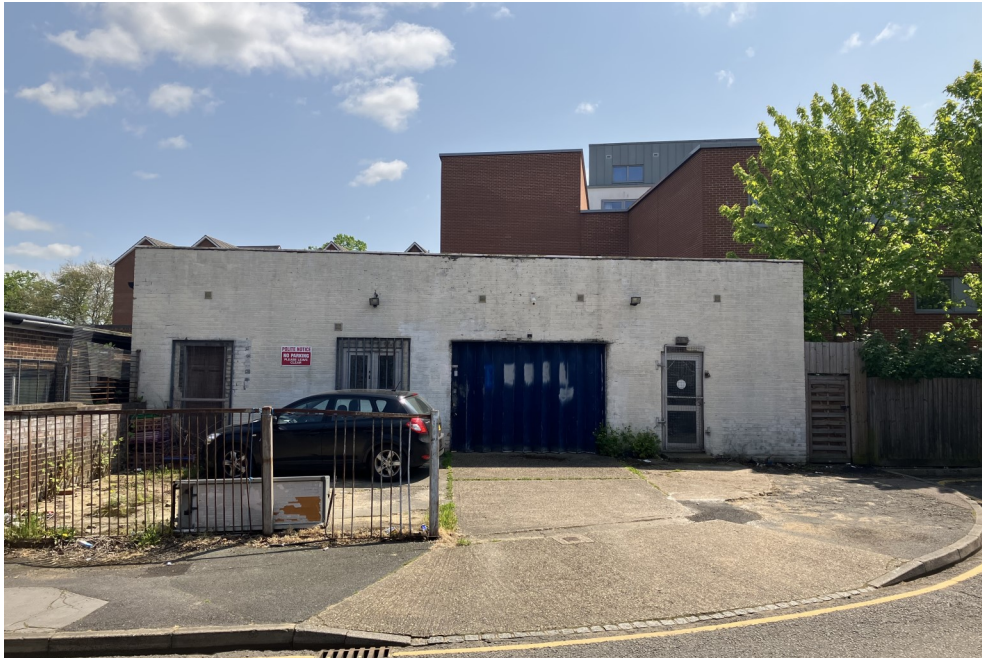
Unit adjacent to rear (southwest) of site
