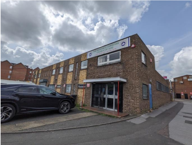
Photo 1: Showing exterior of the front (north) side of building.
