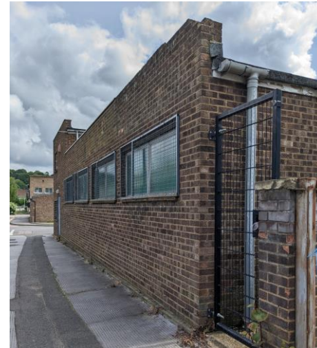
Photo 2: Showing exterior of rear (south) side of building)
