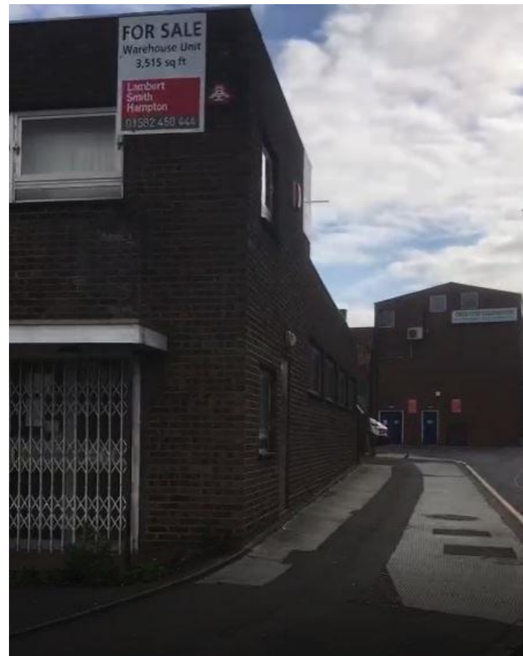
VIEW FROM BOLTON ROAD SHOWING 2 GLOUCESTER ROAD BUSINESS UNIT
