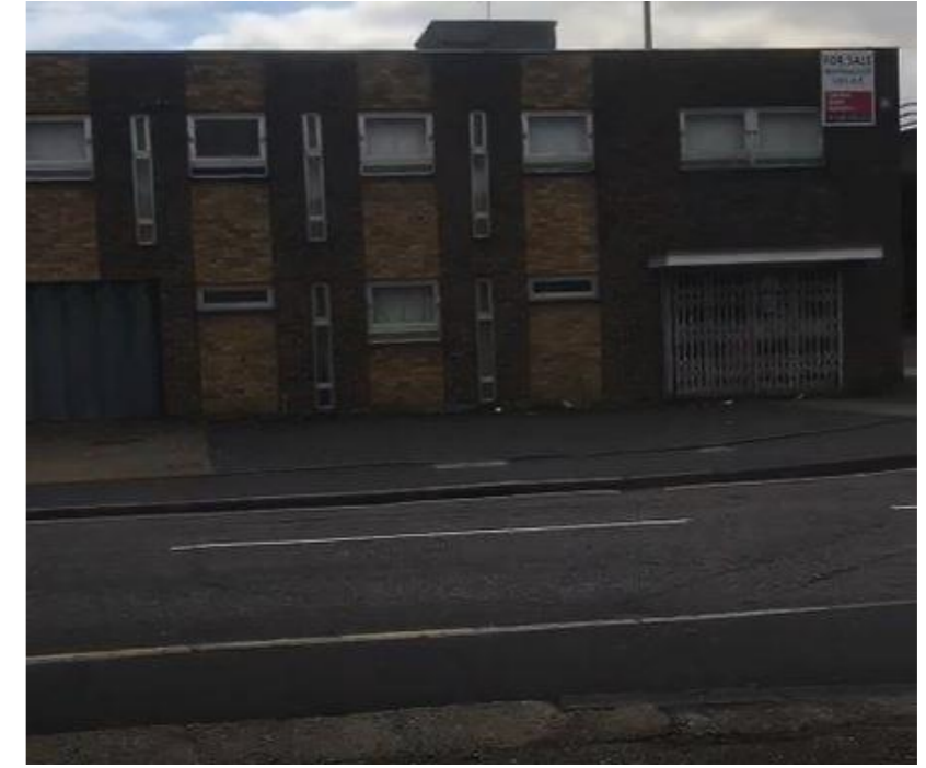
VIEW FROM GLOUCESTER ROAD SHOWING 2 GLOUCESTER ROAD BUSINESS UNIT
