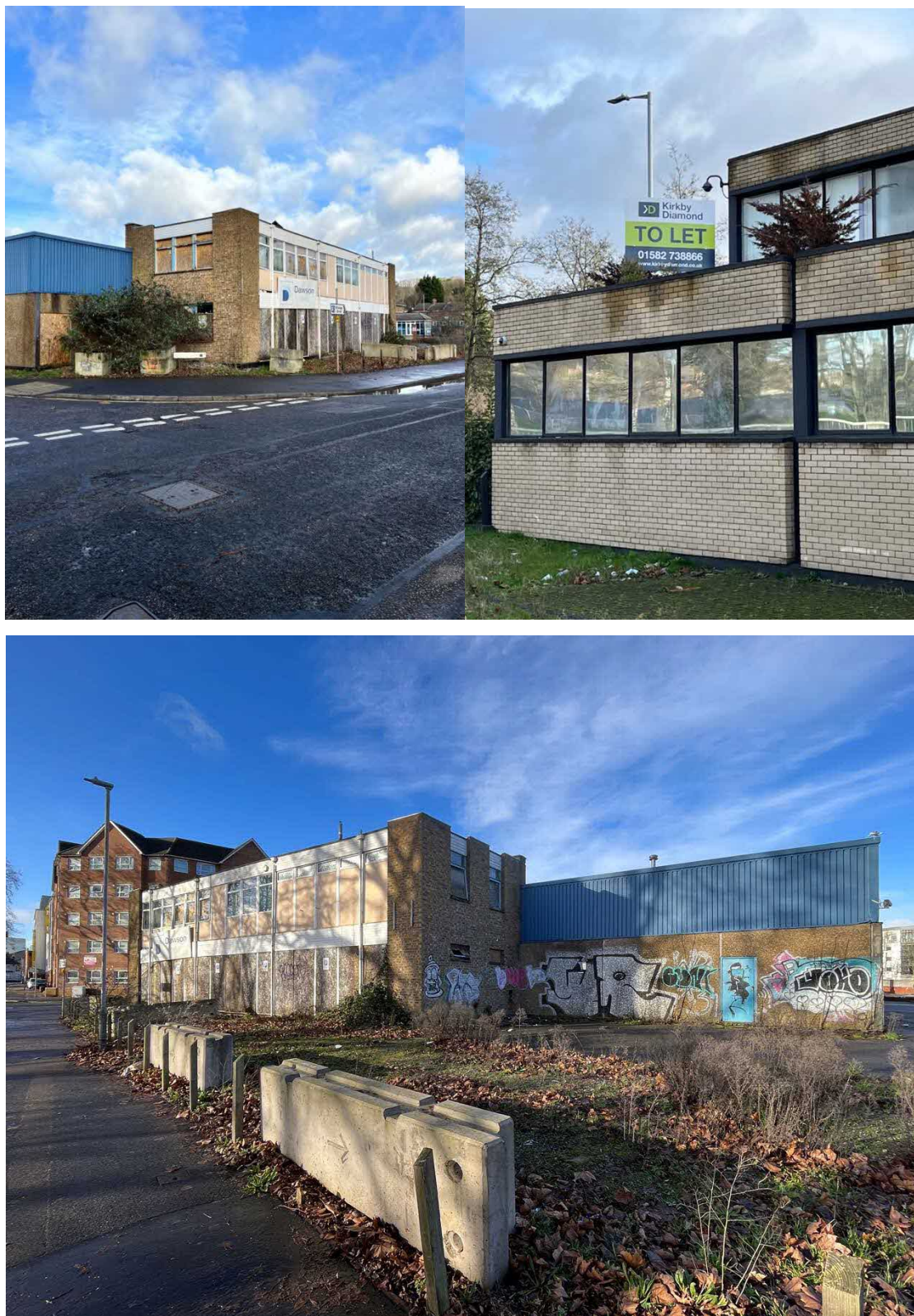
Fig 9. Substantial vacant and/or derelict buildings were noted within 100m of the subject property within the established Category B Employment zone during walkthrough. The zone constitutes an underdeveloped island within a ring of mixed use redevelopment.
