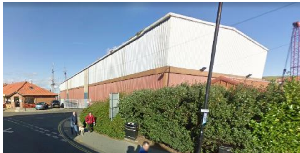
Pre demolition in 2013
