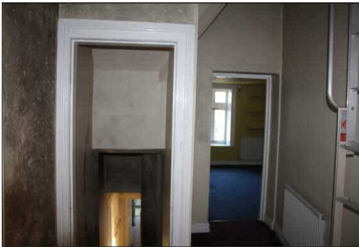
29. First floor landing area (2019)
