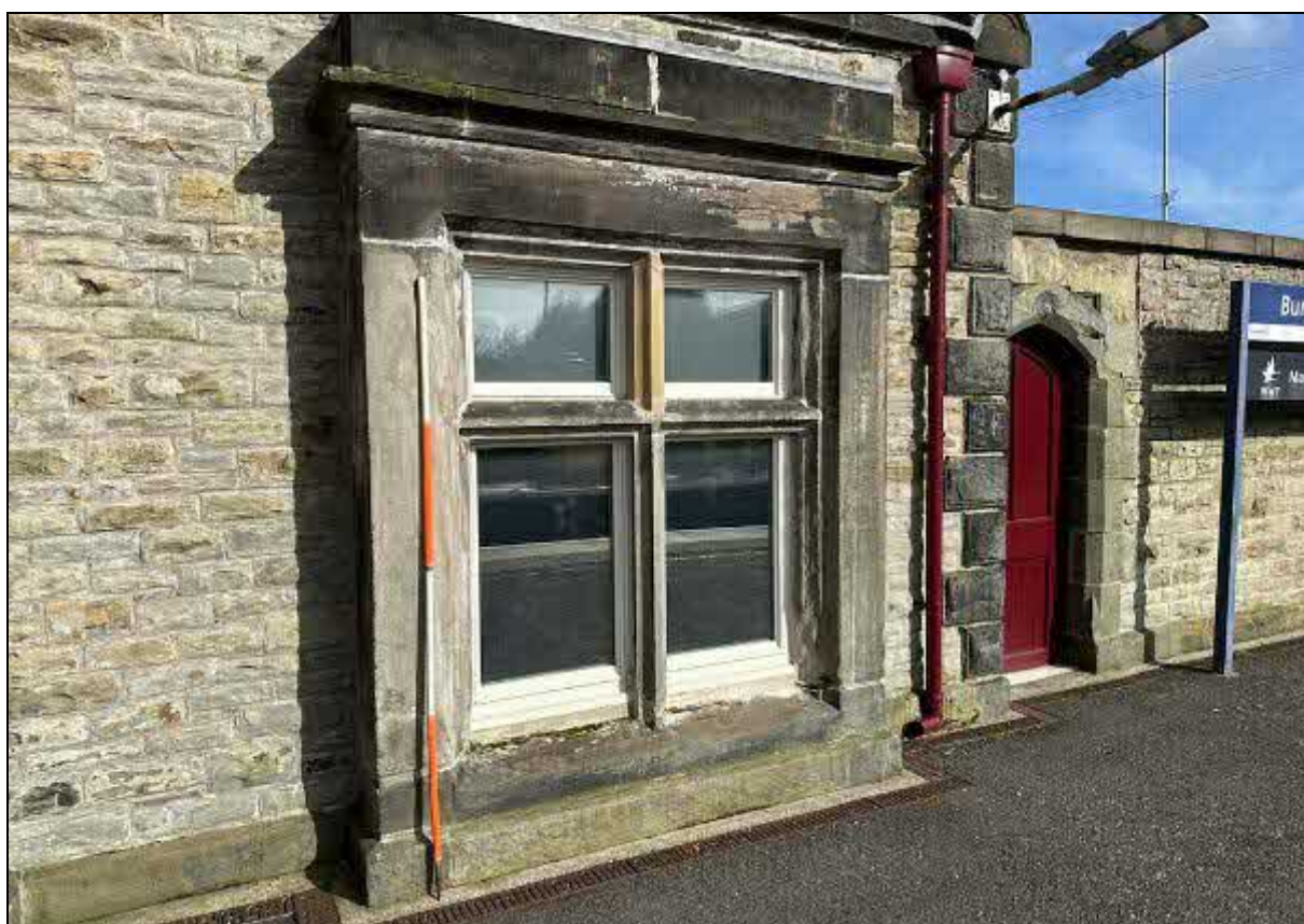
10. Shallow bay at the east end of the front elevation
