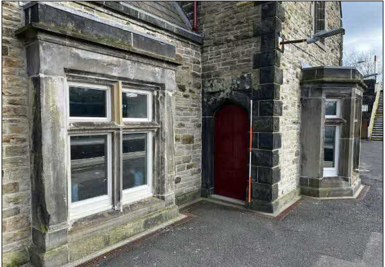
8. Shallow bay window and Tudor doorway in adjoining section
