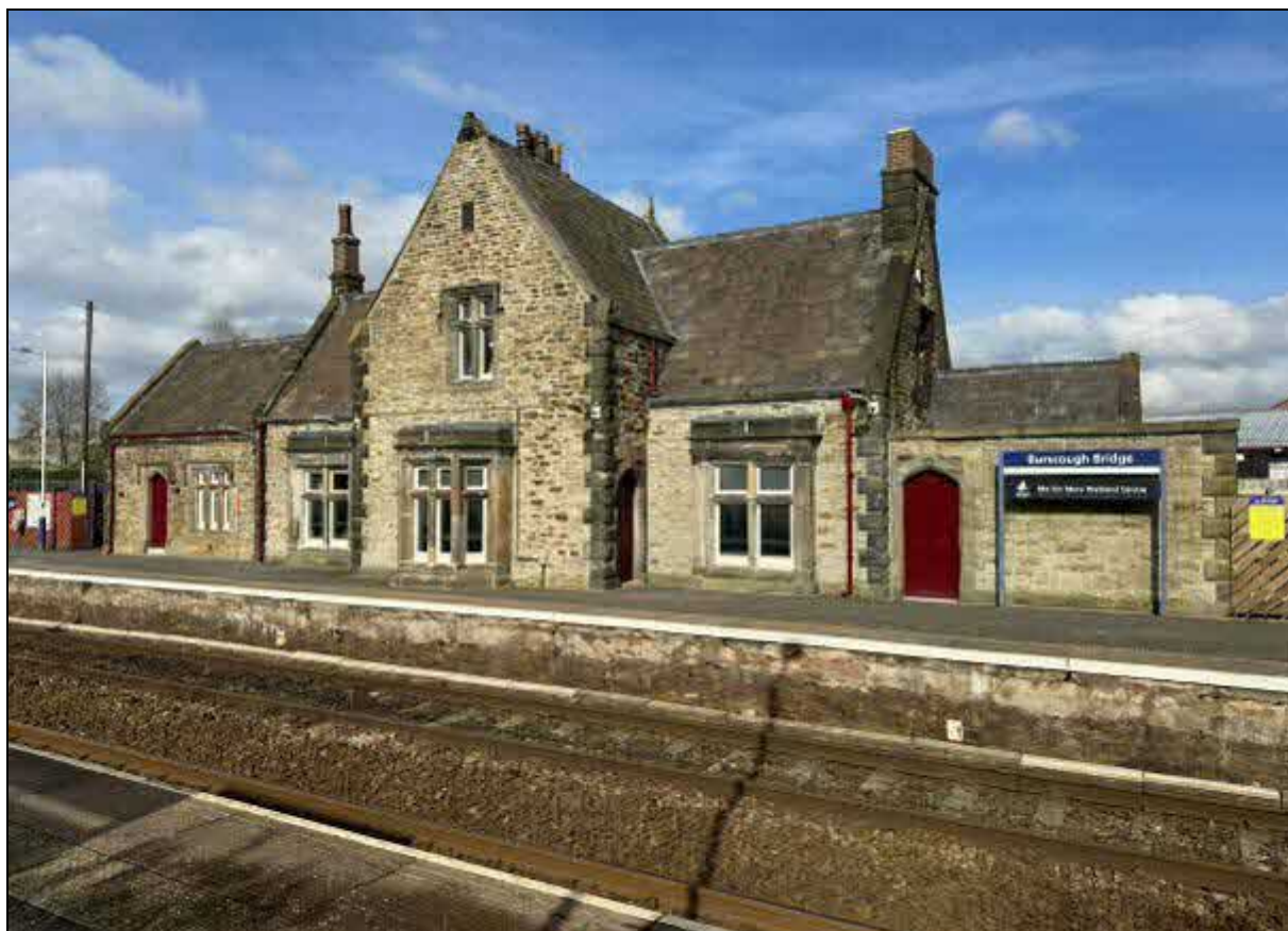
1. The station house: view from the opposite side of the track
