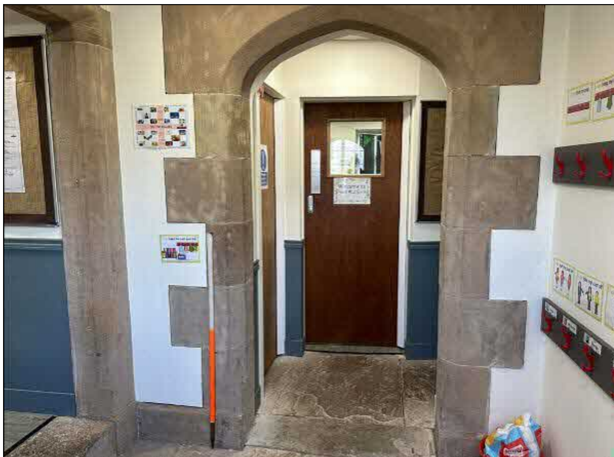
19. Present-day view of lobby in rear porch showing Tudor doorway
