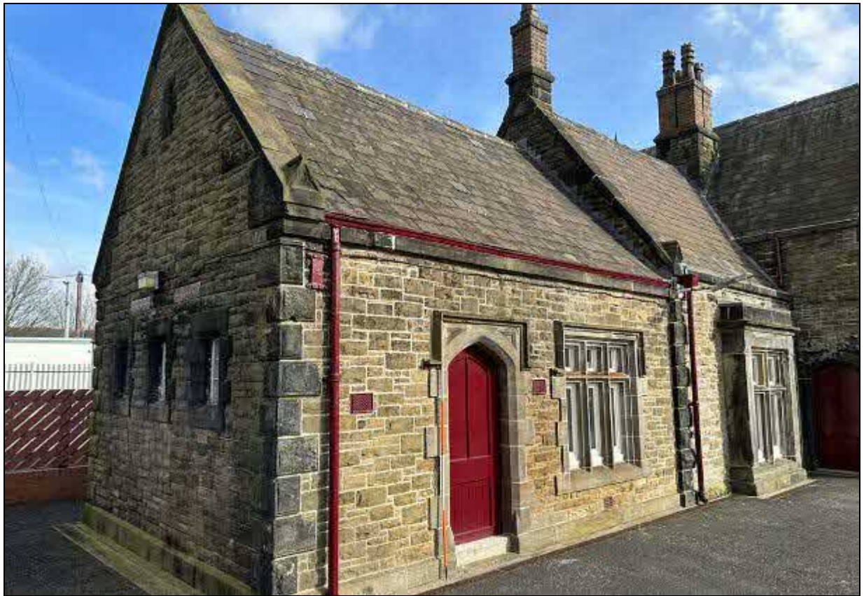
7. Westernmost element of the building: three windows in end wall suggest lavatories inside
