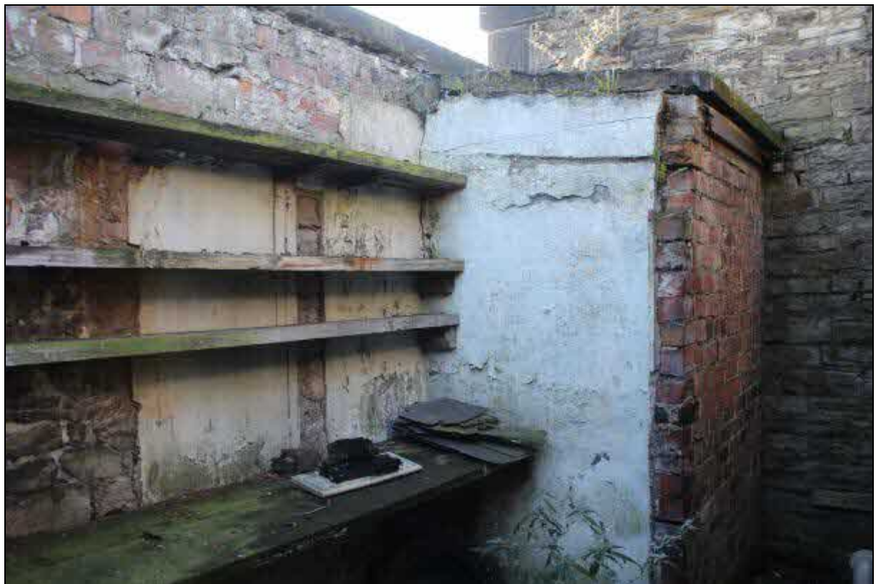
13. Interior of the enclosed yard (2019)
