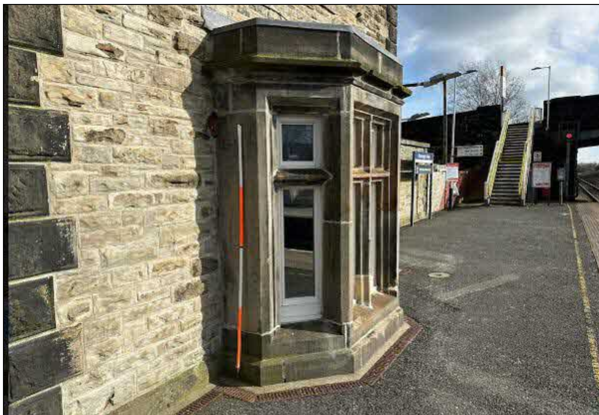
9. Bay window to presumed main waiting room
