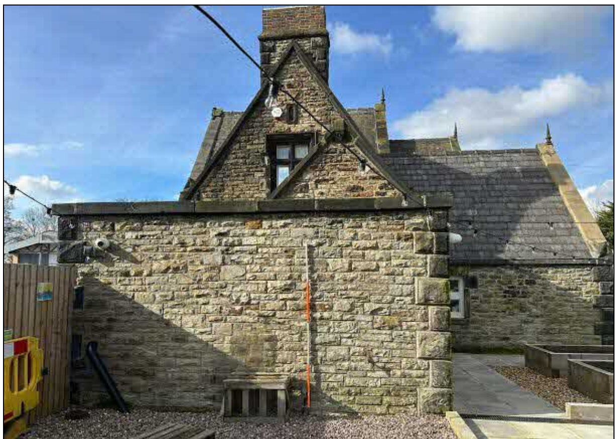
12. View from east showing end wall of enclosed yard
