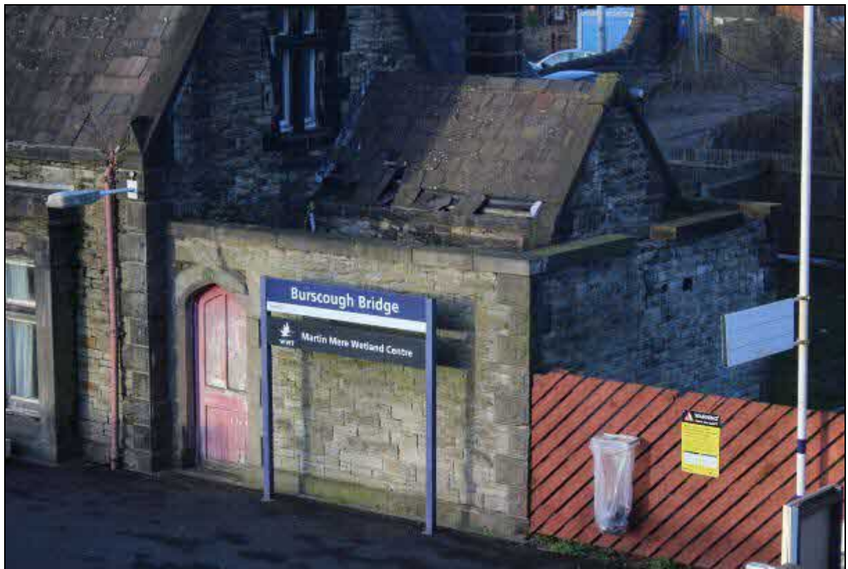
11. View from bridge of enclosed yard and office at east end (2019)
