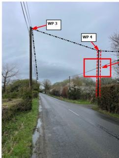
OH WP4 ERECT 1 X 10ML WOODEN POLE WP5 ERECT 1 X 8ML WOODEN POLE WP6 ERECT 1 X 8ML WOODEN POLE WP7 ERECT 1 X 8ML WOODEN POLE
