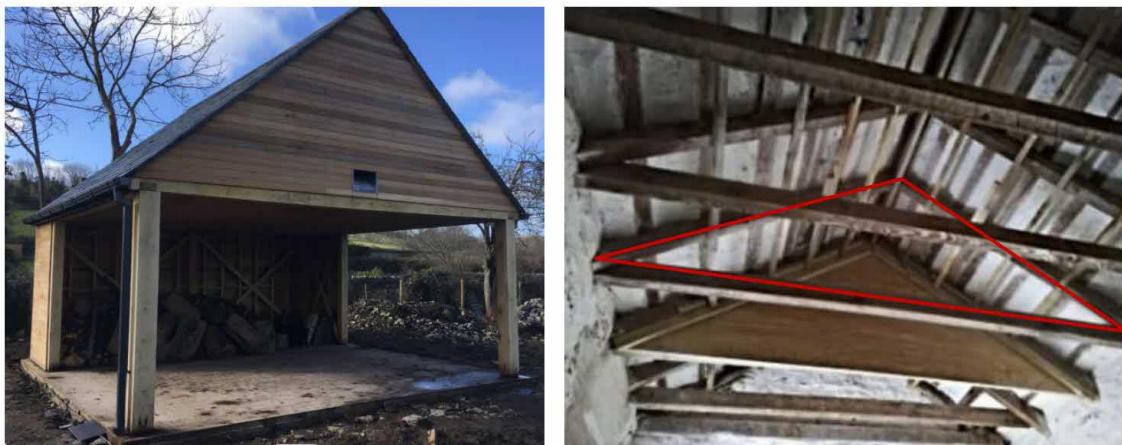
Figure 4: Example of proposed bat house / storage unit and baffle and indicative area for additional baffle to create hot box in roof structure.
