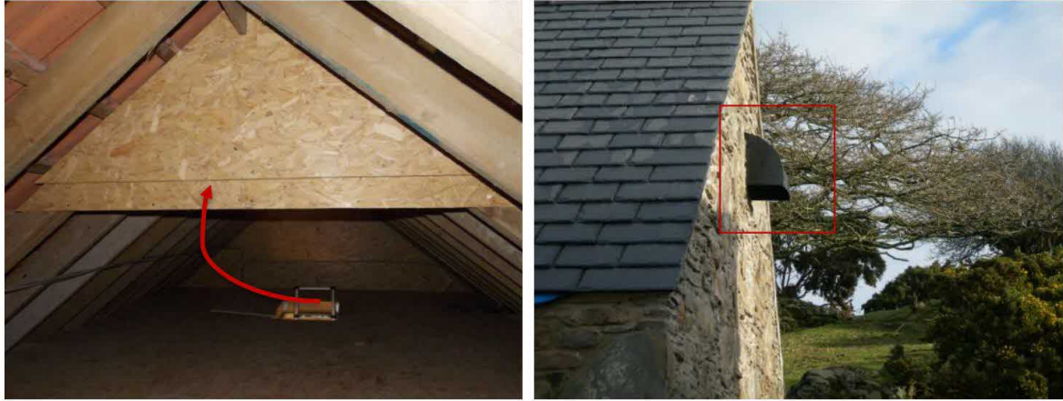
Figure 5: Squeeze box, showing where bat would roost and cowl on exterior of access hole (Chris Hall Ltd Mammal Consultancy, 2012)
