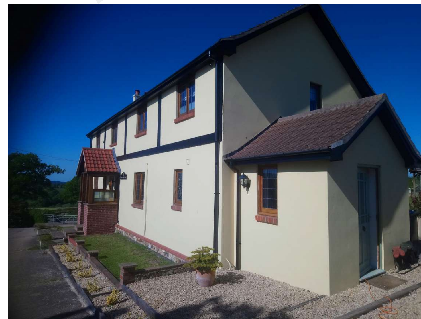
PHOTOGRAPH - EXISTING HOUSE ASPECT - Arrow B
