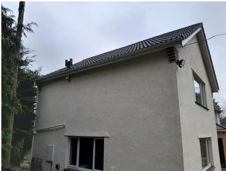
Photo 3. Eastern elevation of the dwelling
