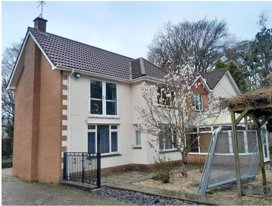
Photo 2. Rear of the dwelling looking north east
