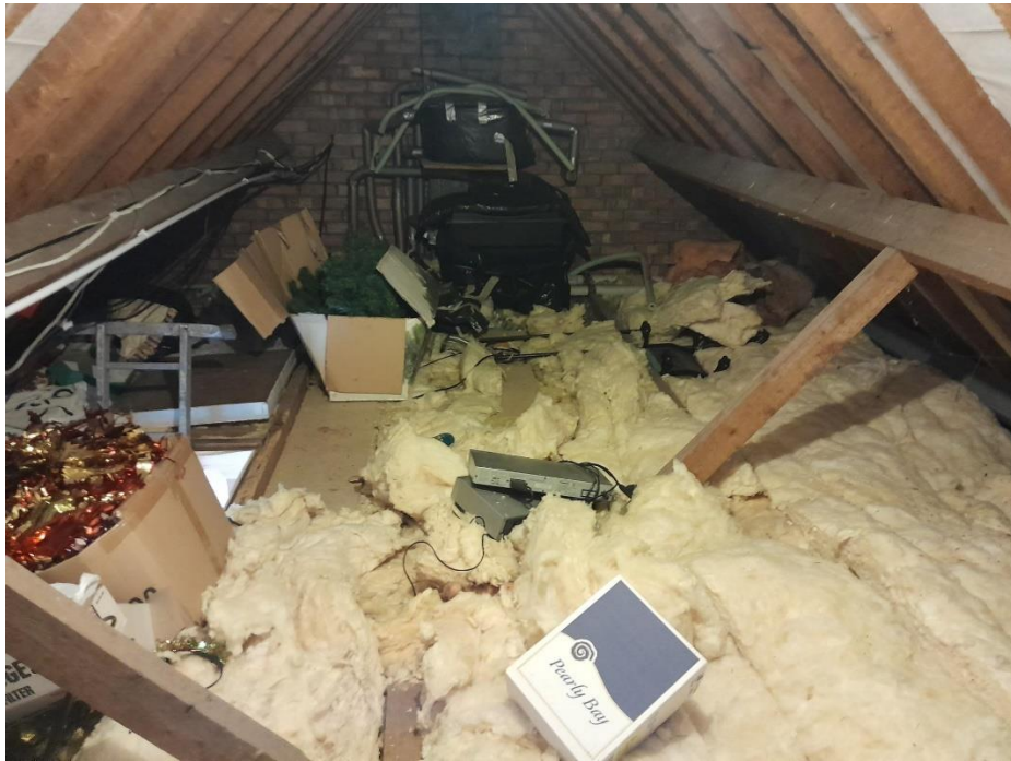
Photo 6. Internal roof space – Void B
