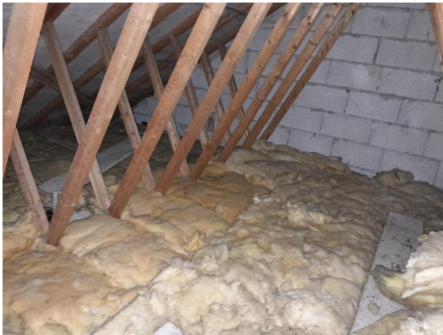
Photo 5. Internal roof space - Void A
