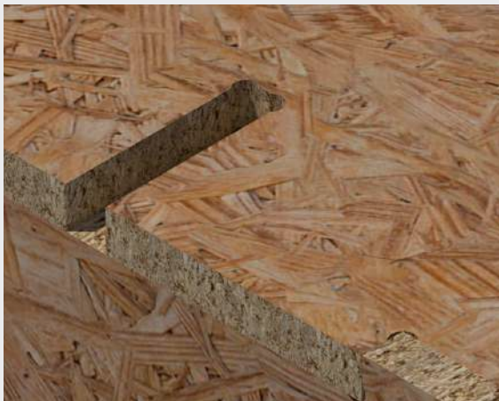
Peg connection cut-outs. CNC timber pegs locate and align the faces of cassettes on site prior to nail plates fixing.
