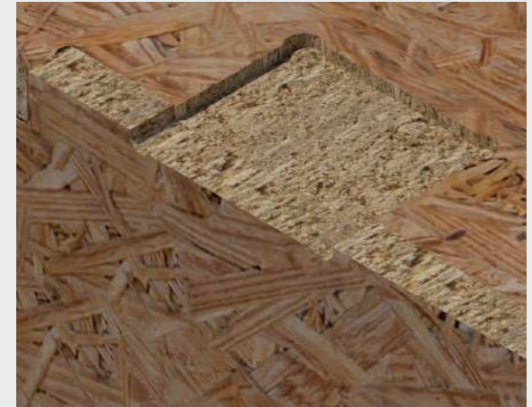
Rebated areas for nail plate fixing, ensuring that engineer's fixing spec is adhered to on site at all times.
