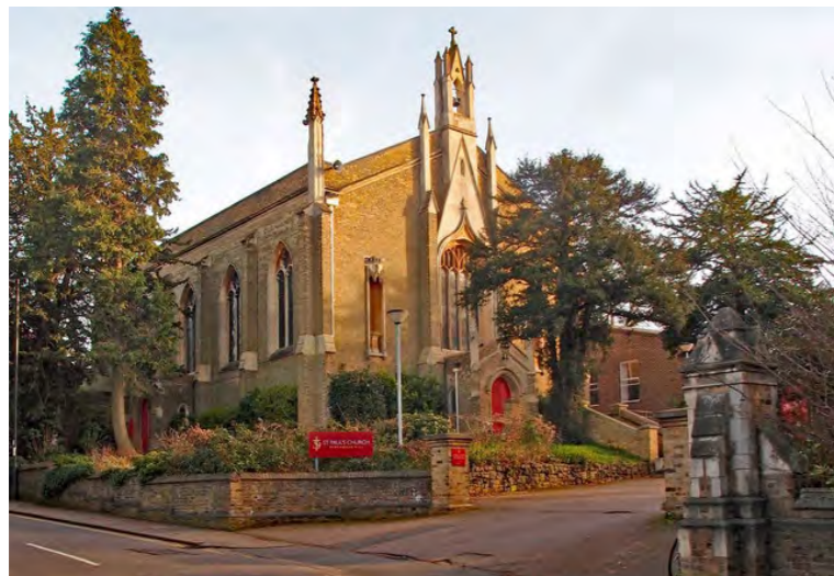
Entrance with most posts and railings no longer in situ, notice the stepped stone wall on the roadside has been lost
