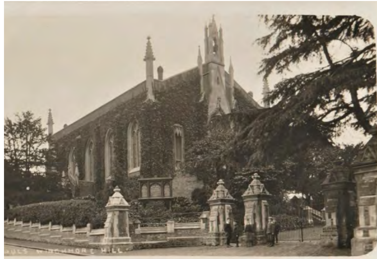
Historic buttressed posts with pedestrian and vehicle access with iron railings and gates
