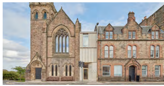
Greyfriars Charteris Center, by Konishi Gaffney Architects
