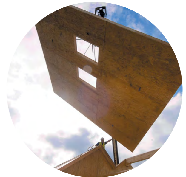
Off site construction
