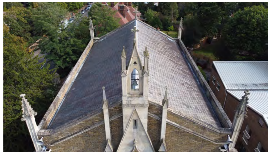
A view of the roof and single bell
