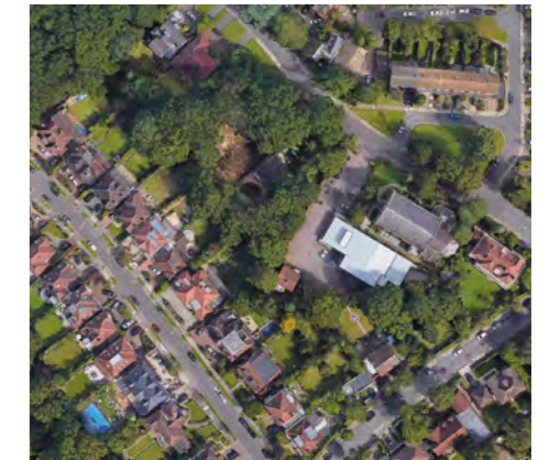
Modern aerial view, showing school demolished (carpark)
