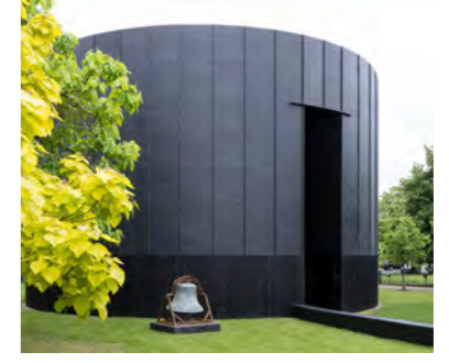
Black Chapel by Theaster Gates Serpentine Pavilion 2022
