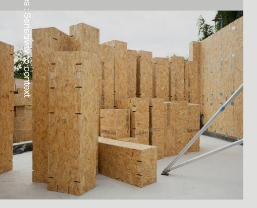
The BlokBuild system is not only much quicker and safer than traditional methods of construction, it also requires fewer operatives on site. For 56a Church Hill we estimate an installation duration of 4 weeks, with a 4-person team.
