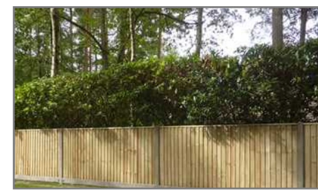
1.2m Close board fence with badger proof mesh at base
