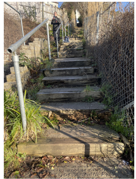
Photo of footpath steps and block wall
