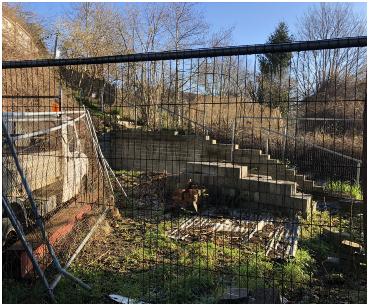
Photo of site showing block wall and footpath steps behind
