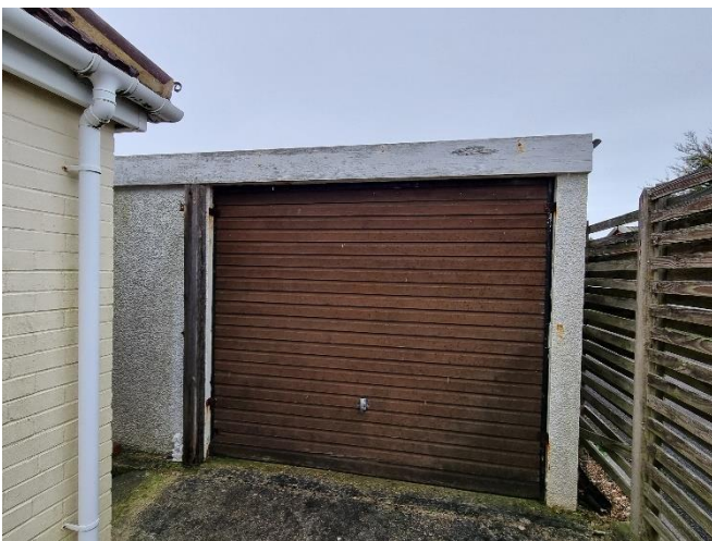
Photo 1: West facing elevation of garage
