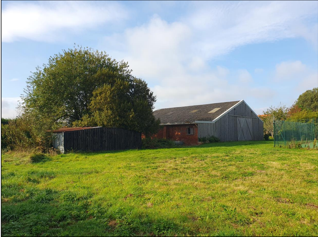
Northern elevation of existing agricultural barn
