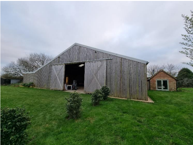
Photo 3: North facing elevation of barn.
