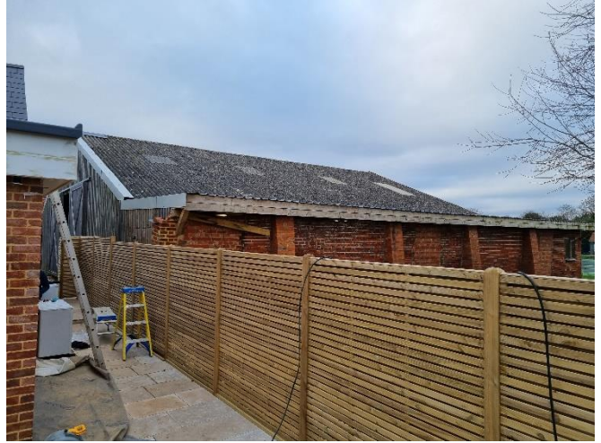
Photo 2: East facing elevation of barn.
