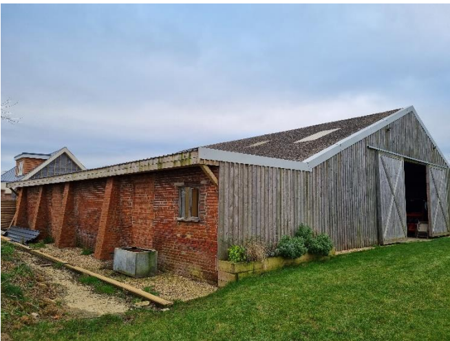
Photo 5: North east corner of barn.
