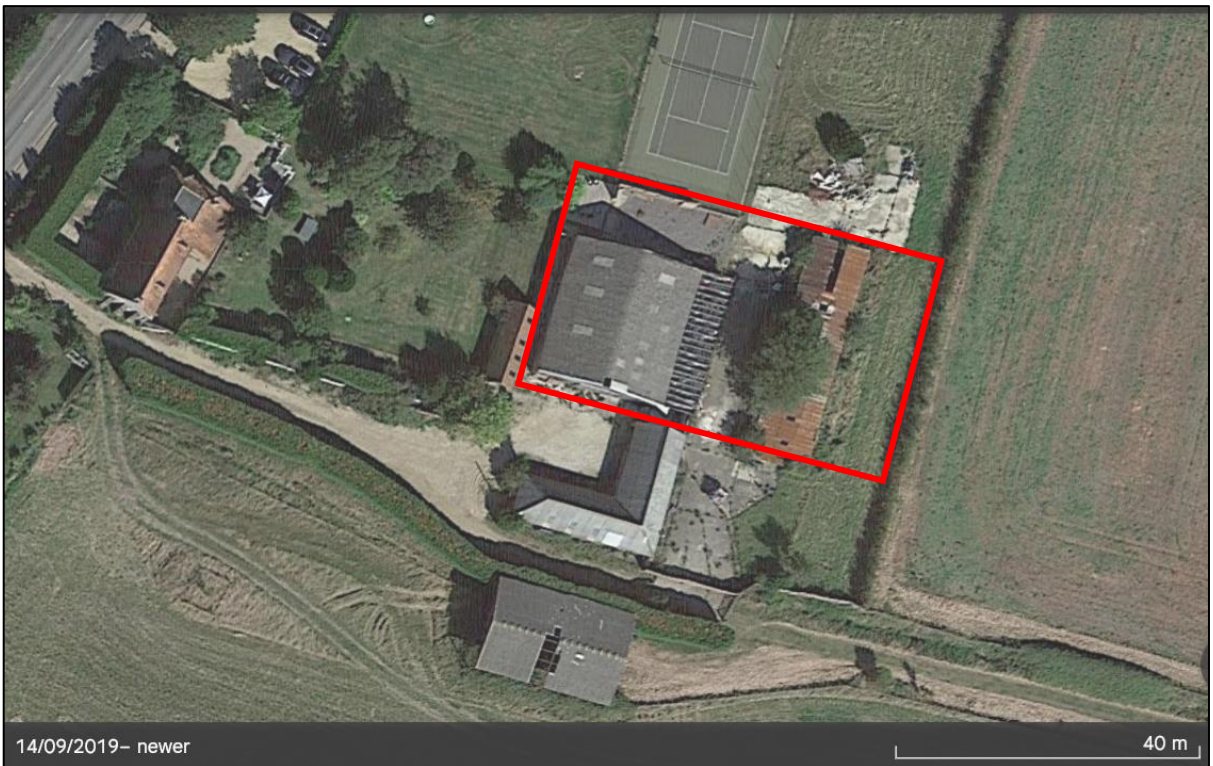
Figure 2 – Aerial view of site with red line boundary. ©Google Earth 2024
