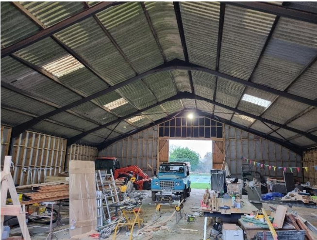
Photo 13: Interior of barn.
