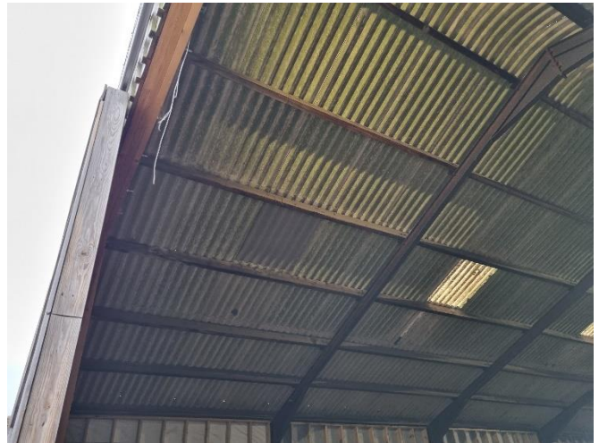
Photo 14: Interior roof of barn.
