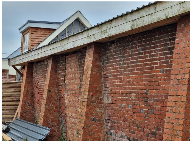
Photo 6: Brick section of barn.
