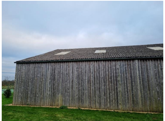
Photo 4: West facing elevation of barn.
