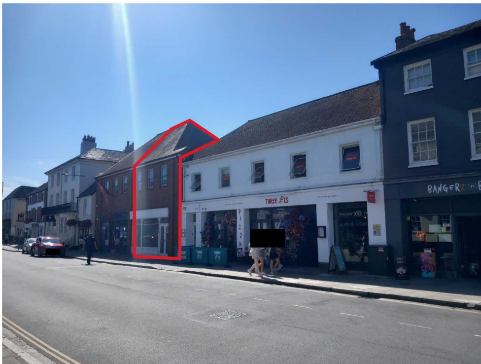
Front elevation viewed from the north
