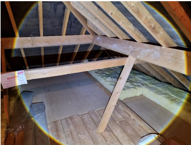
Photo 3: Interior loft void
