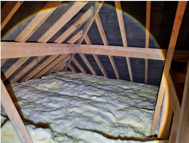
Photo 1: Interior loft void
