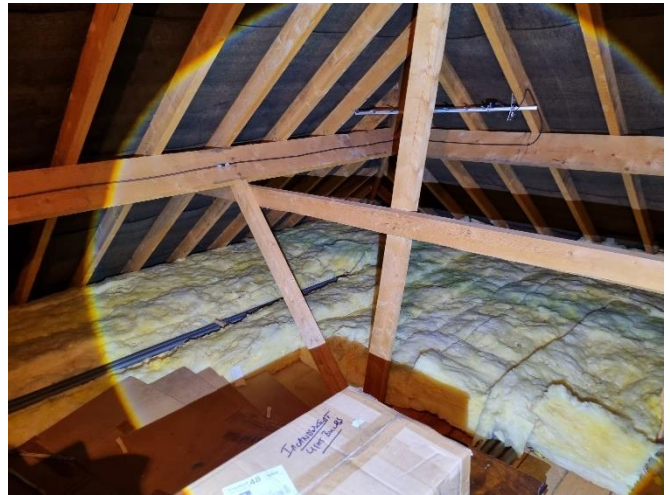
Photo 2: Interior loft void
