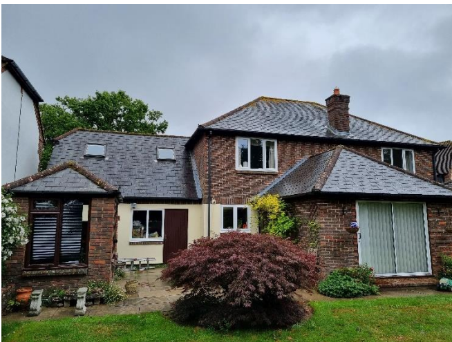
Photo 5: West facing elevation
