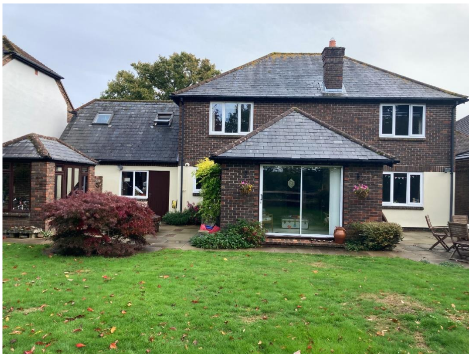
Image-2 Showing rear of the existing property.
