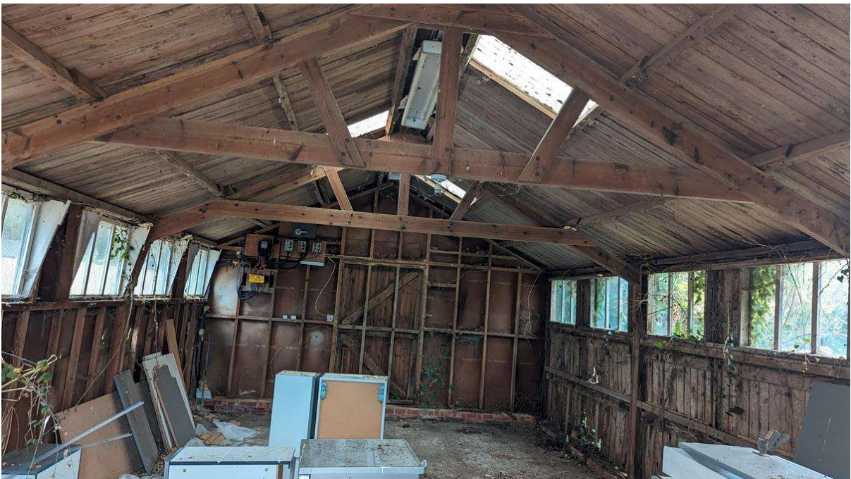
Photo 4 – View inside B2.
