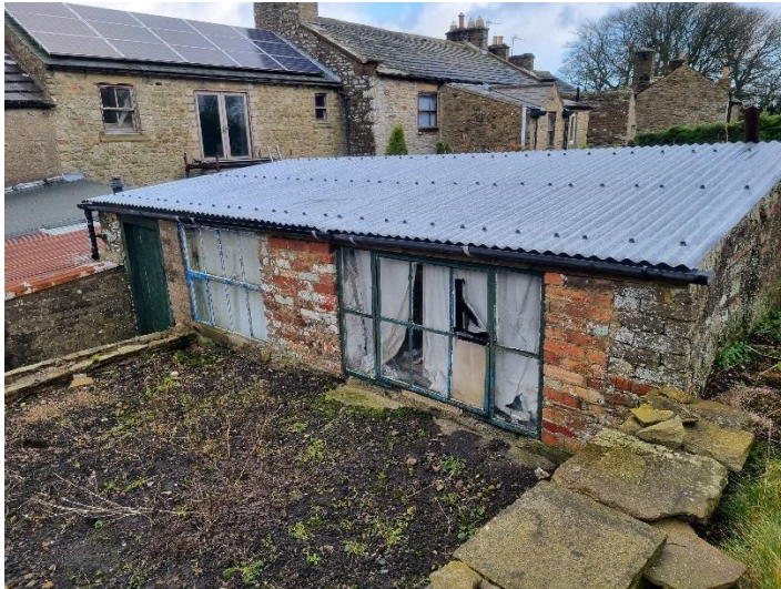
External store – profiled zinc cladding.
