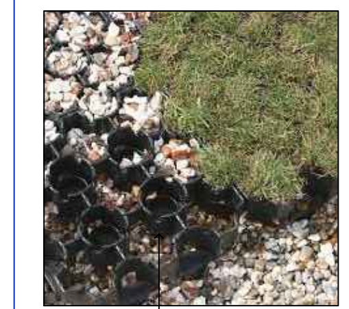
PARKING / TURNING AREA: PODPAVE 85 C/W GRASS INFILL
