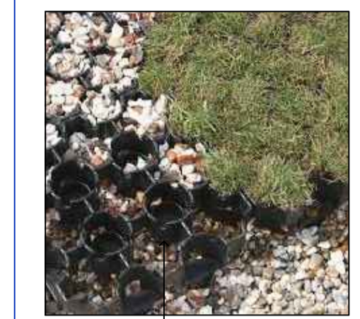
PARKING / TURNING AREA: PODPAVE 85 CW GRASS INFILL
