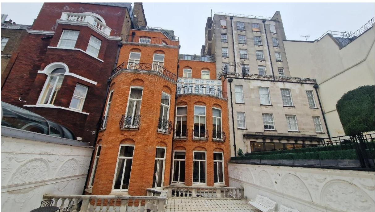
Rear elevation as it exists today.
